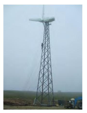
TDX Power completed the design and procured materials, equipment, labor, permits and supervision to construct a fully operational 65 kilowatt Wind Turbine Generator System (WTGS) and associated equipment and interconnect to the newly commissioned diesel fuel based power plant in Nikolski in accordance with the International Electrotechnical Commission (IEC) Wind Turbine Standards. This was accomplished by July 28, 2007.
