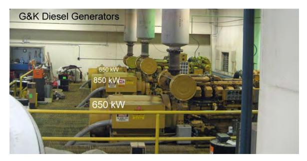
The generators were installed in 1987 and now have between 67,000 and 79,000 hours of operation on them. The generators are well maintained and each one has been rebuilt at least twice. G&K expects them to have a usable life of 150,000 hours. Replacement cost for a single generator is over \$300,000. Below is a summary of the generators and their status.
