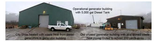
During the site visit an old waste heat recovery system was found at the Old Generator Building that includes a 3" HPDE piping loop to the school approximately 200 yards away. The pipe was insulated with spray foam only on the top side of the piping, with no other protection from the environment.
