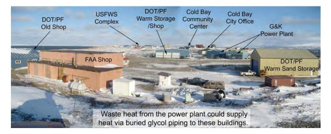
The buildings in each scenario will receive heat from an insulated, buried district heating loop that delivers waste heat from G&K's diesel generators. Piping lengths vary depending on the scenario. Please refer to the Moolin report for piping lengths, building heating loads, waste heat production and system layout.
