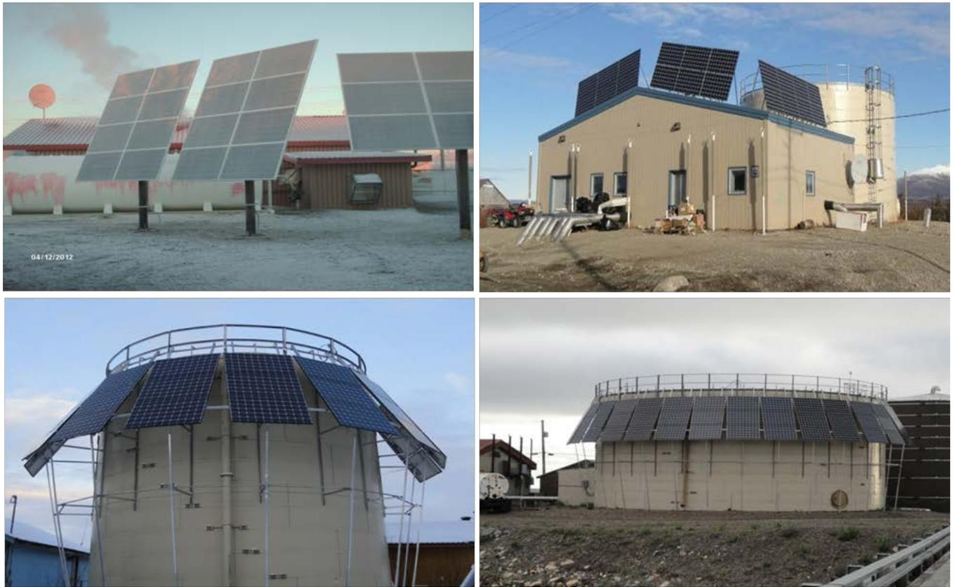
**Figure 3. Solar PV installations at water treatment facilities in the remote villages of Ambler, Shungnak, Deering, and Kobuk, Alaska<sup>6</sup>**
