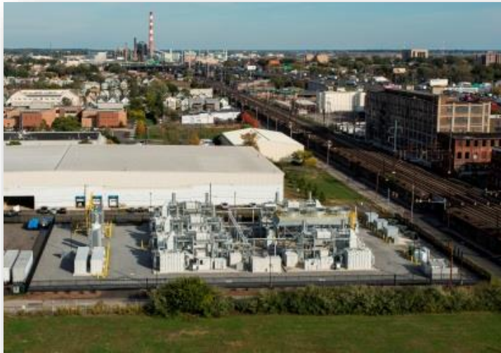
14.9 MW fuel cell park Bridgeport, CT
