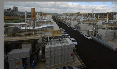
59MW fuel cell park
