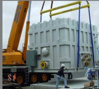
Completed module 1.4 megawatts
