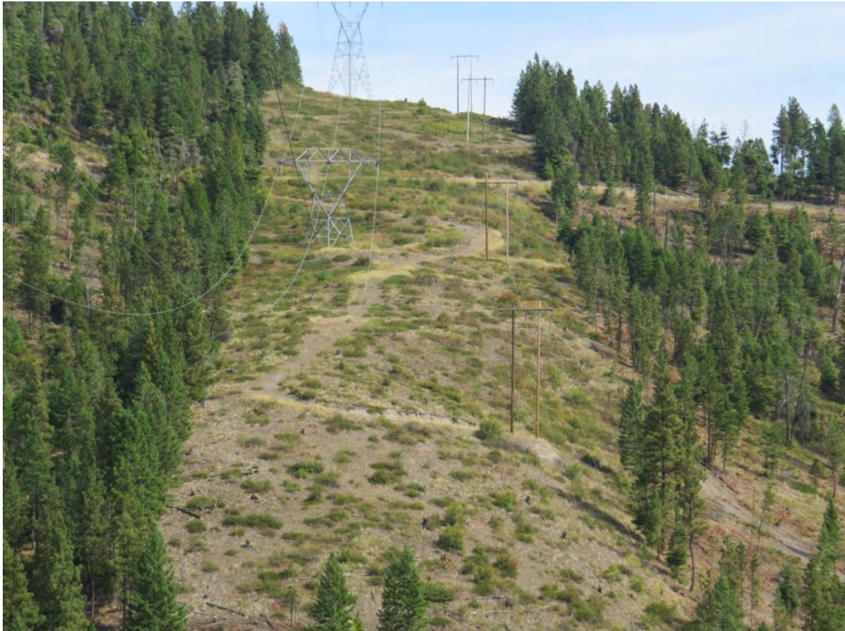
Figure 3.3-1. Looking North at Line Mile 20: Steep Slopes, Exposed Bare Ground, and Gravel Access Road Switchbacks Across the Transmission Line Right-of-Way
