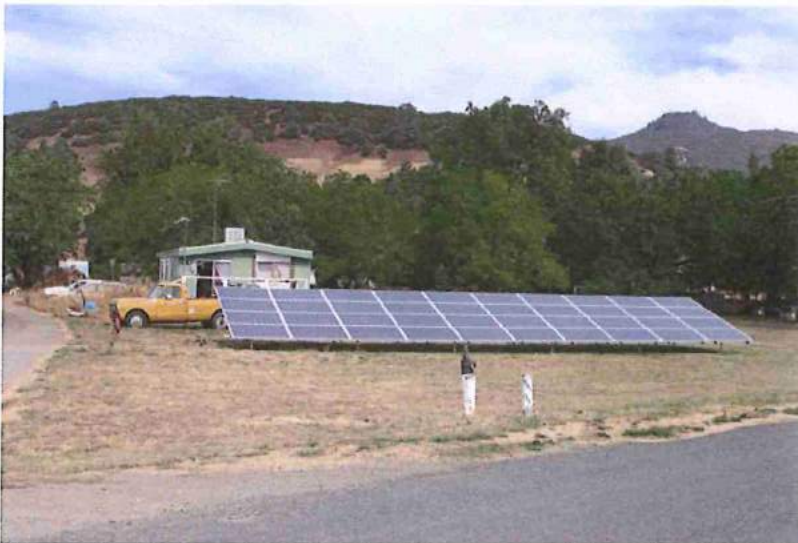
Figure 22. A ground mounted solar array providing electricity to a Tribal home in Lake County, California. The ground mounted system was used due to poor roof orientation and ease of reconnection to a possible future replacement structure.
