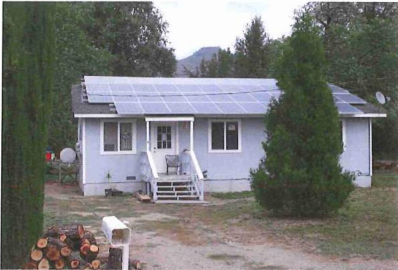
Figure 21. A roof mounted solar array providing electricity to a Tribal home in Lake County, California. In this case, the array is servicing two homes providing a significant savings for installation.
