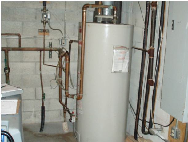
Figure 69. The domestic water heater (left).
