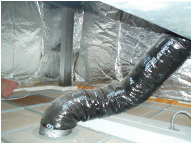
Figure 41. The foil-faced fiberglass insulation continues on the wall below the roof until it intersects the wood framed wall where the drop ceiling begins (left).
