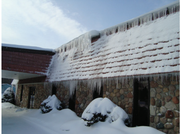
Figure 58. An example of a large sheet of ice beginning to shed off the roof (right). Sliding snow and ice should be considered as part of the structural analysis for a PV system.
