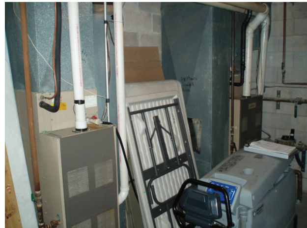
Figure 70. The recommended location for the solar thermal storage tank is in between these two furnaces (right). Currently this space is used for general storage of folding tables and other supplies. The water heater is approximately 10 feet away and is located just to the right of the photo edge.
