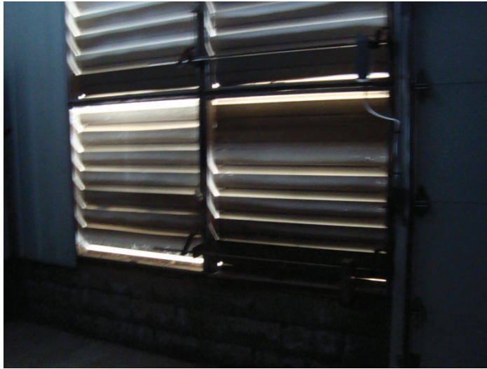
Figure 26. Leaky generator building intake dampers.
