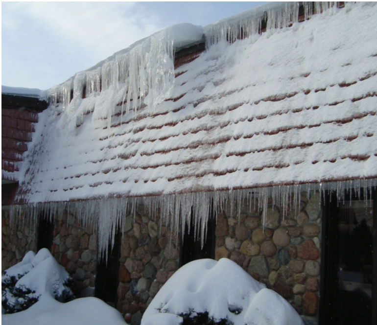
Figure 44. Ice damming near the east side entrance adjacent to car canopy
