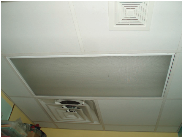
Figure 20. The exhaust grille for a bathroom fan can be seen in the top of this image (left).
