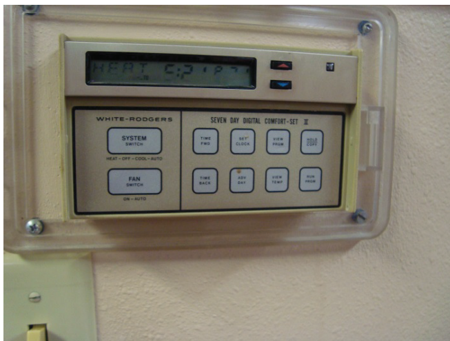
Figure 31: Lobby thermostat LCD screen is failing.
