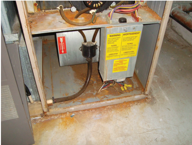
Figure 26: Gym furnace unit with missing filter. Filter is typically installed at the connection between return duct and the fan section.
