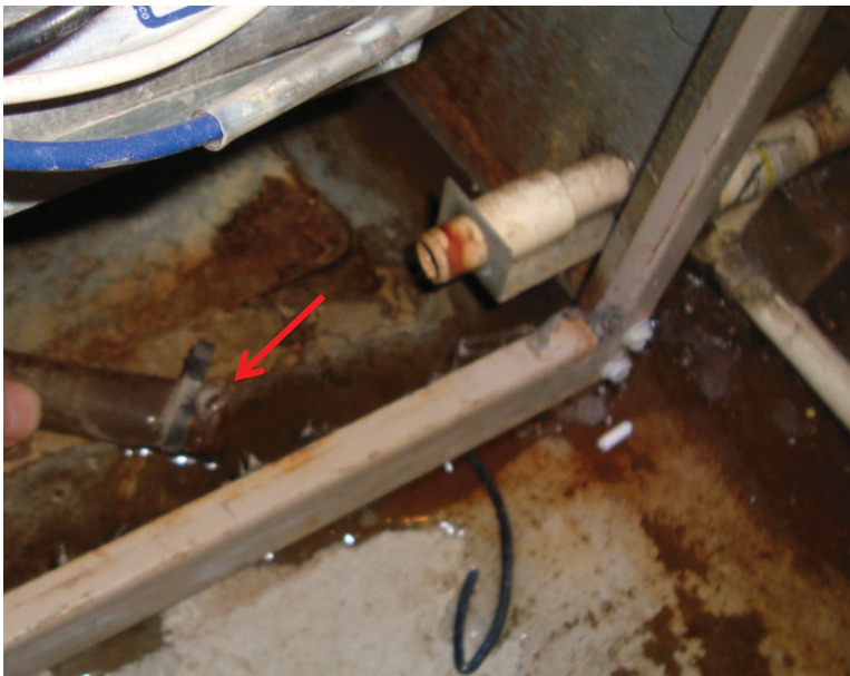
Figure 25: Condensate hose was disconnected from the PVC drain.
