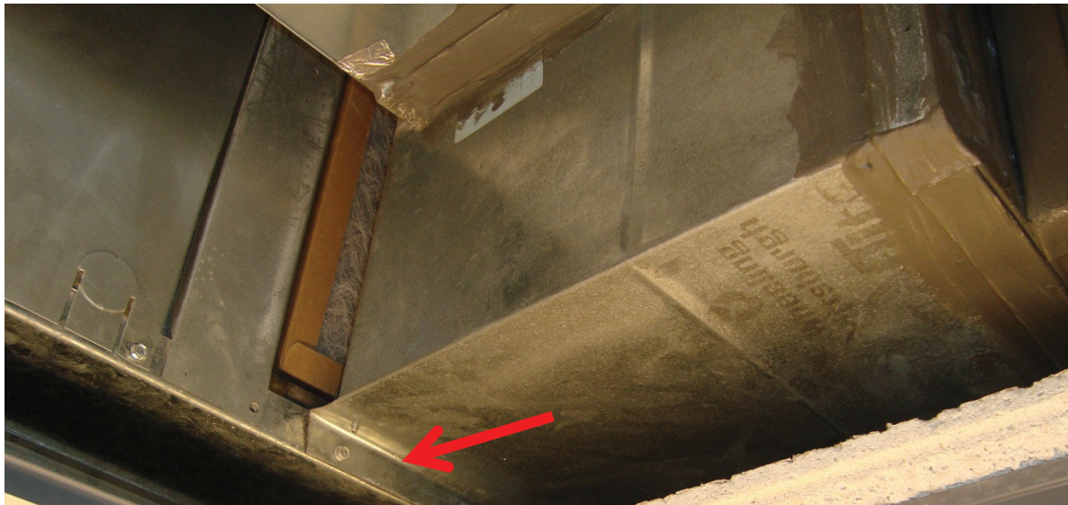
Figure 17. Connection of return duct to heat pump without a flexible connection between the heat pump and duct causing noise issues.
