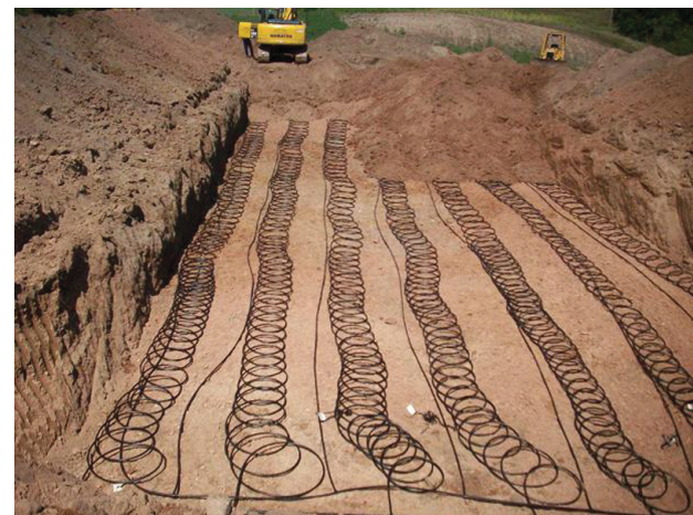
Figure 46. A typical racetrack horizontal loop geothermal field (left). This field served a 10,000 ft 2 fire station in Madison, WI. Figure 47. A typical slinky horizontal loop geothermal field (right). Photo credit: G.O. Loop, Randolph, WI.
