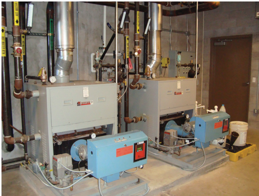
Figure 14. The heat pump loop boilers.
