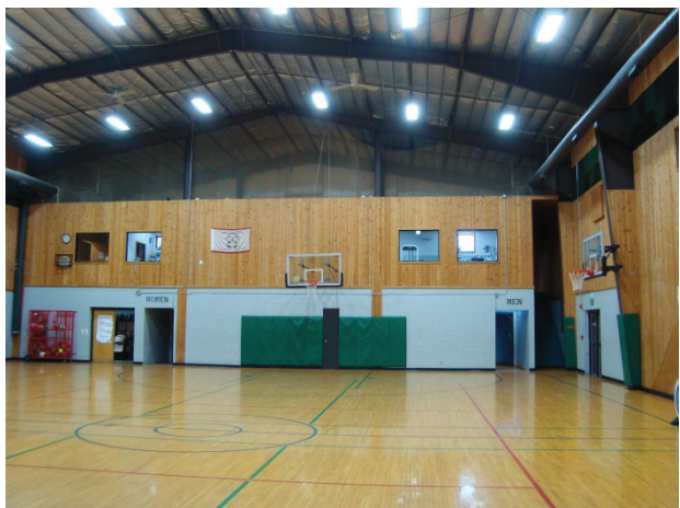
Figure 68. A view of the roof structure (right). The main beams and purlins can be seen in this photo.
