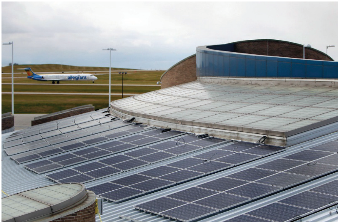
Figure 56. A photo of a typical PV system on a roof type that is similar to the metal roof on the MFC.
