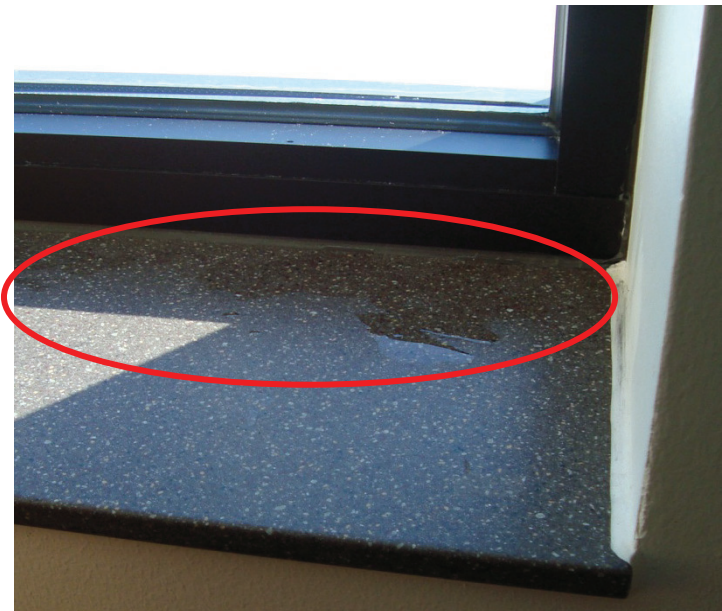
Figure 23. Condensation on the window sill from cold window frames.
