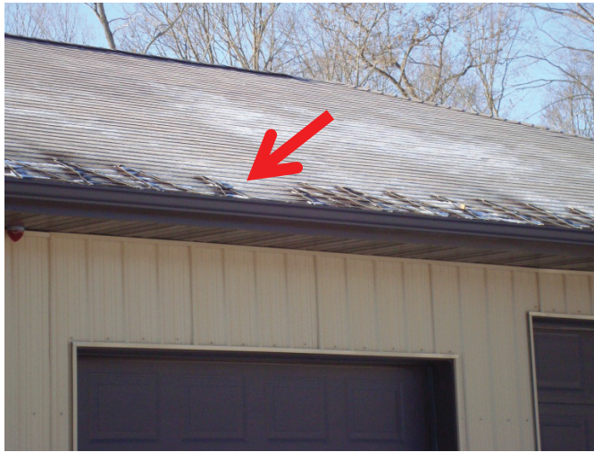
Figure 27. Heat trace heating but there is no risk of ice damming.
