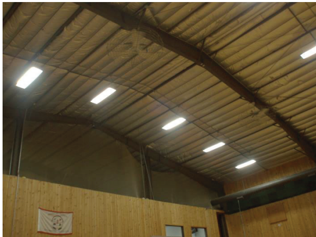
Figure 39. Foil-faced fiberglass roof insulation in the gym (left).
