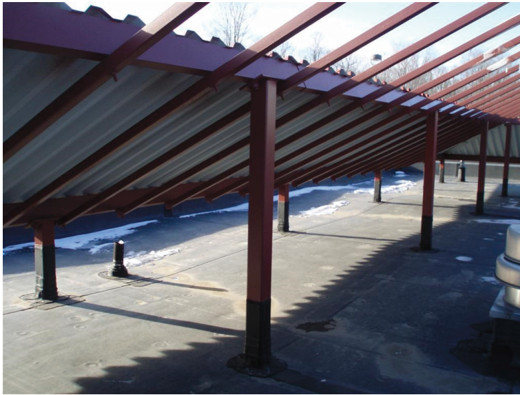
Figure 35. A photo showing the structure supporting the architectural panels. The architectural panels are attached to a C-channel that spans across square tubing pedestals that penetrate the roof and are welded to the steel I-joists. The observed areas of this structure appeared to be in good shape. The paint was intact and no rust was seen. A structural engineer should be consulted to determine the structural adequacy for use with solar electric or solar thermal collectors.
