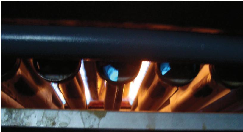
Figure 16. AHU-1 duct furnace flame pattern.
