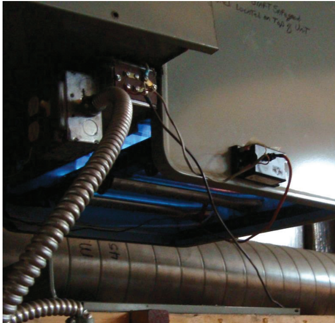
Figure 30: West gym unit burner cover removed and is sitting directly below unit.
