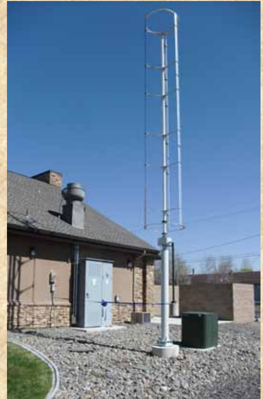
Dresslerville Community Center
