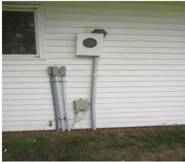
Figure 3: Existing and unused metering infrastructure at the four-plexes
