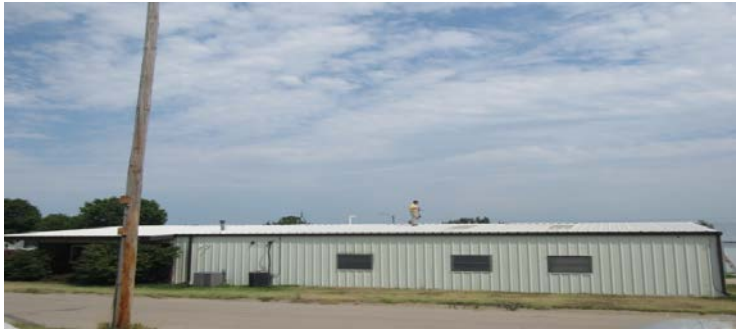
Figure 3: The HQ Building looking from the South, note outside condenser location.
