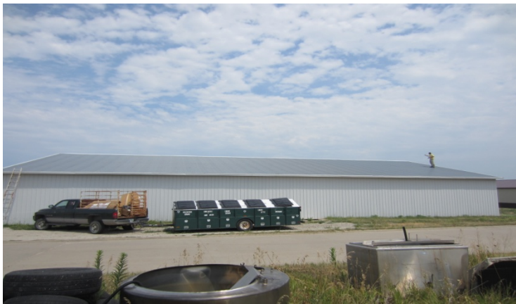
Figure 4: Maintenance garage building from the south, note exceptional solar roof.
