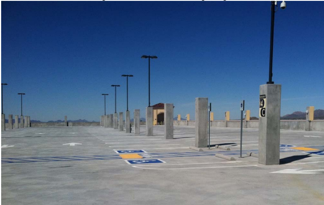
Figure 33: Casino Del Sol Parking Garage
