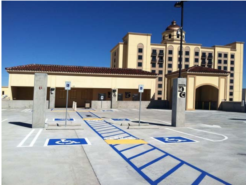
Figure 34: Casino Del Sol Parking Garage
