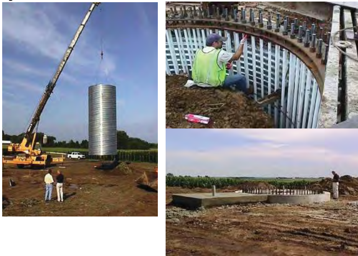
Figure K-1 – Post Foundation
