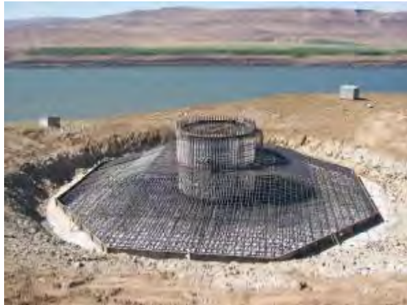
Figure K-2 – Spread Foundation
