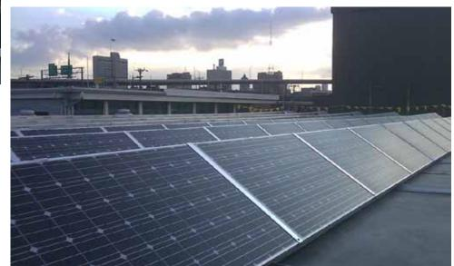
Step Four - The solar panels feed their solar electrical energy into an inverter which converts it from D.C. power to A.C. power and in turn feeds this power to the building for consumption
