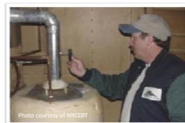
Test for draft above the draft diverter.
