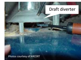
On start up, time the amount of spillage. Then test draft above the draft diverter. Spillage should not exceed 1 minute.
