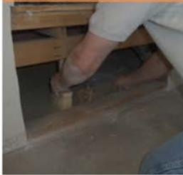
Line plenum with duct board. Mechanically fasten duct board to framing.
