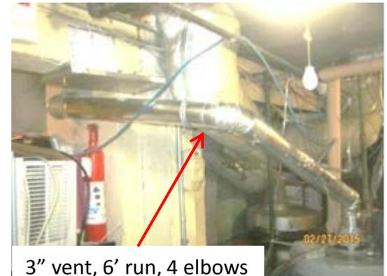
> WI\_01 had a large opening downstream of the water heater (unused, partially repaired connection for a furnace)
