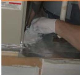
If refrigerant and condensate lines terminate to the outside, install hardware cloth or equivalent rodent barrier.
