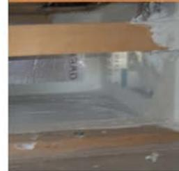
If refrigerant and condensate lines penetrate the platform return, provide infill and seal as needed.
