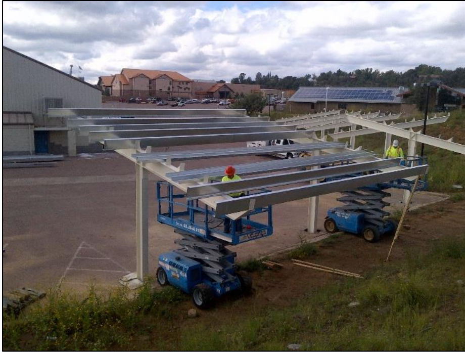
Erecting canopies in gymnasium parking lot
