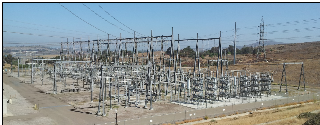
Figure 2-14. Example of a 230-kV substation.
