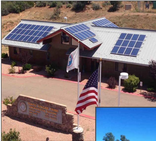
Tonto Apache Tribe Solar photovoltaic systems installed on their government buildings (AZ)
