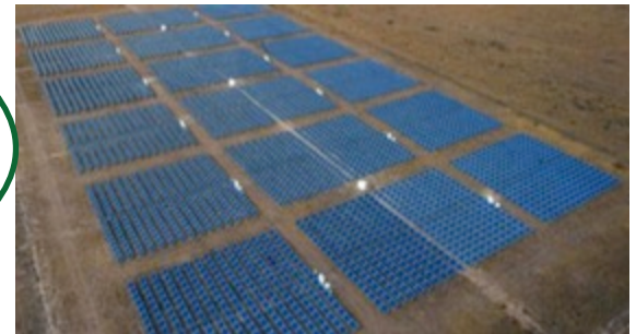
Tucson Electric Power, NREL 13327
