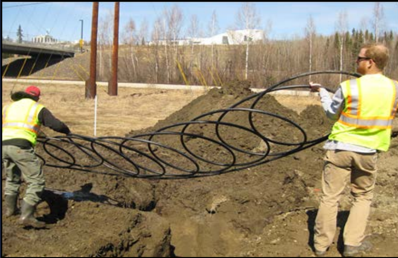
Installing cold climate heat pump
