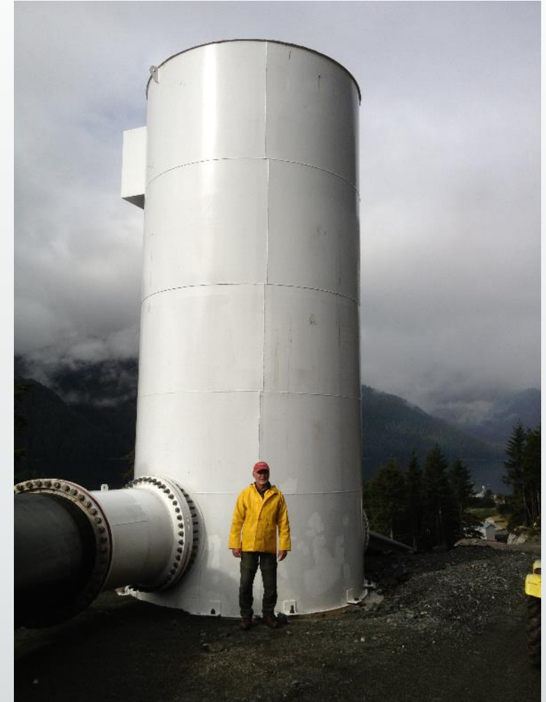
Pelican surge tank
