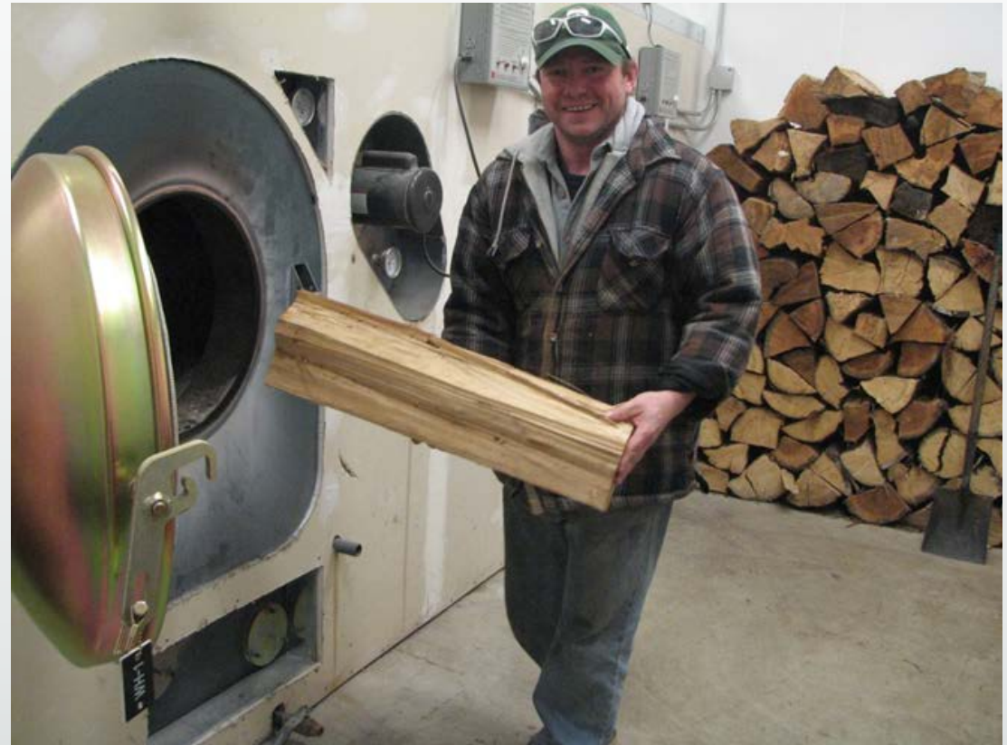
Coffman Cove School Garn boiler.
