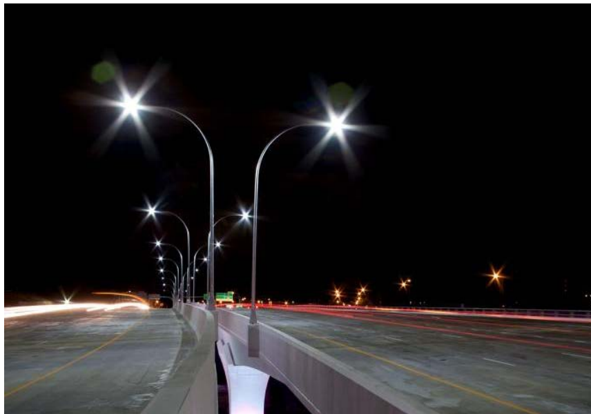
Figure 2. LED luminaires on the I-35 bridge
