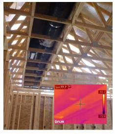
Attic chase and infrared image taken during a winter heating cycle
