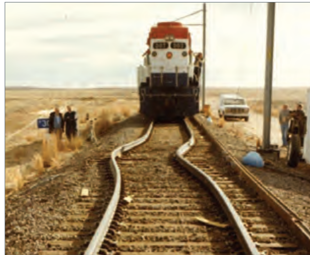
Figure 2-9. Rail Thermal Misalignment 135
