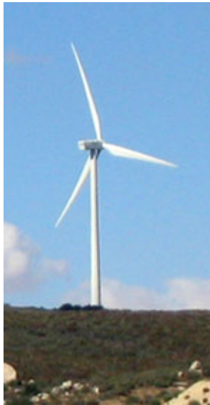
The 25MW Kumeyaay Wind Farm At Campo Reservation
