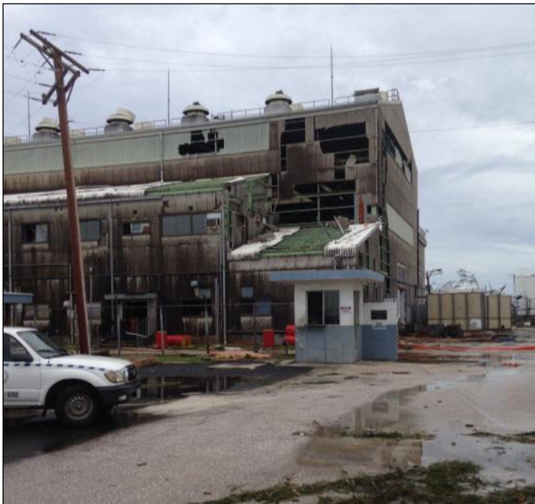
Damage identified to the Commonwealth Utility Corporation's (CUC) 70 MW diesel-fueled power generation plant located in Tanapag, Saipan brought on by Typhoon Soudelor. Photo taken August 3, 2015. Photo credit: ESF-12 DOE Responder Embedded with FEMA IMAT Team on Saipan. Source: U.S. Department of Energy
