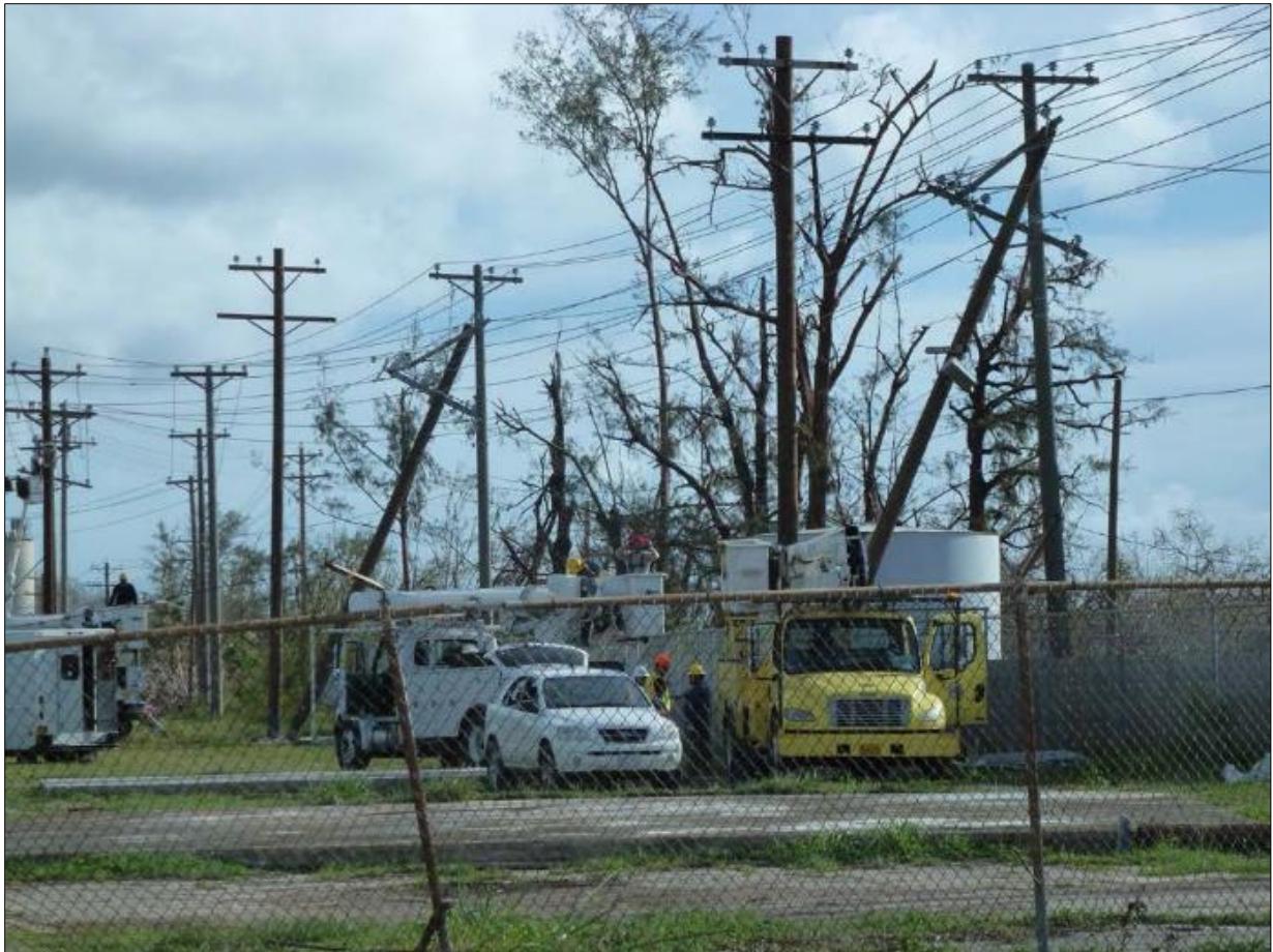
CUC and GPA crews repairing distribution lines in Saipan following damage from Typhoon Soudelor. Photo credit: ESF-12 DOE Responder embedded with FEMA IMAT. Source: U.S. Department of Energy.
