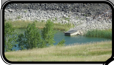
Water retention structures on the site. The structures are some of the measures used to slow drainage off the site and prevent erosion and flooding.
