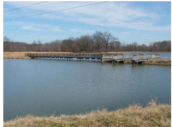
A portion of the former Paducah site buffer area is now used as a wildlife preserve in KY.
