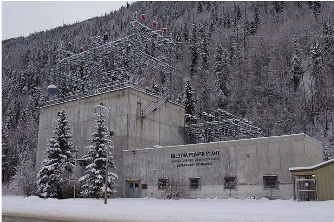
The Eklutna Hydroelectric Power Plant in Alaska, formerly part of the Alaska Power Authority, was sold in 1998.
