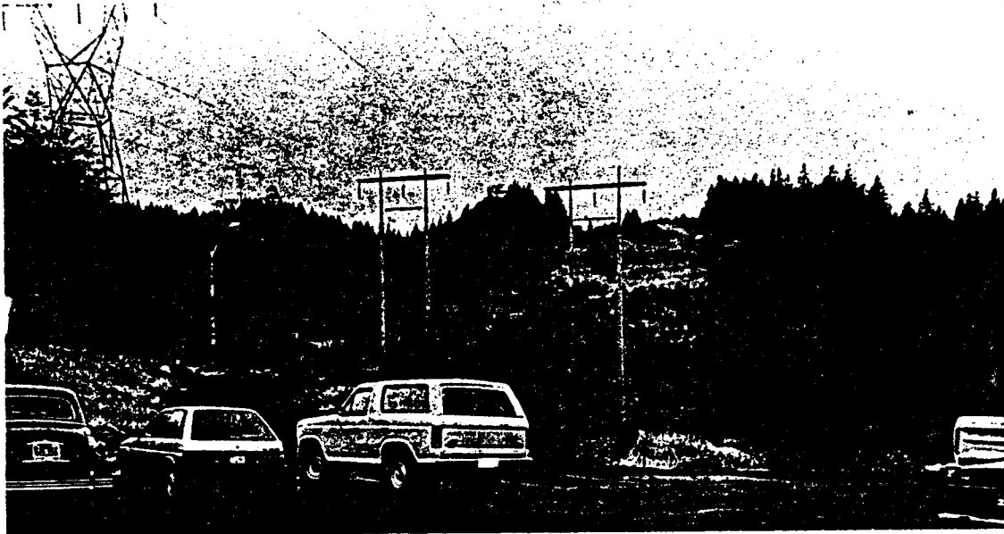
a. Existing view, looking west from the parking lot of an apartment complex near the intersection of Donald Street and Fox Hollow Road. The existing right-of-way has 230-kV steel lattice structures and two 115-kV H-frame, wood pole structures.
