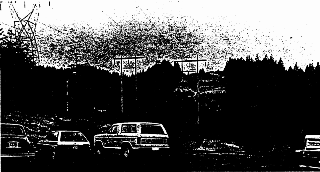
c. Existing view, looking west from the parking lot of an apartment complex near the intersection of Donald Street and Fox Hollow Road. The existing right-of-way has 230-kV steel lattice structures and two 115-kV H-frame, wood pole structures.
