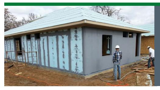
Sterlingbrook Homes installed a sheathing of R-5 rigid EPS foam board over the studs. For bracing at the corners, R-3 rigid foam was installed over half-inch OSB. A water-resistant membrane was sprayed over the foam and took the place of house wrap to provide a weather-resistant air barrier. Inside, the wall cavities were filled with open-cell spray foam for a total wall insulation value of R-21 to R-23.
