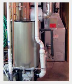
This photo shows a combi system replacement using a condensing storage water heater and a hydronic air handler. At this home, this system saved more than 20% on space and water heating natural gas usage.
