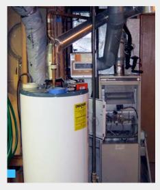
For existing systems in the basement of a single-family home, space heat was provided by a forced-air natural gas furnace with an AFUE rating of 78%. Water heating was provided by a natural draft natural gas water heater with an EF rating of 59%.
