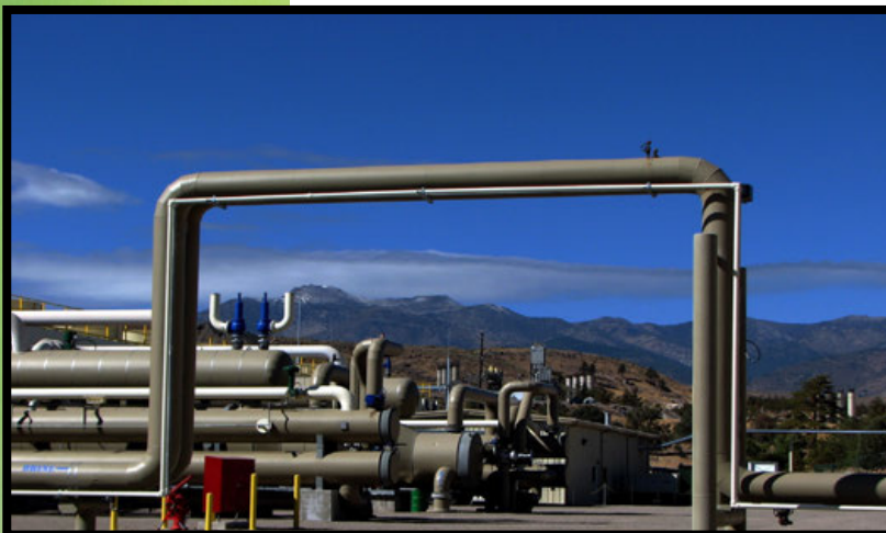
Galena power plant, part of the Ormat Steamboat geothermal complex in Nevada. Source: GRC
