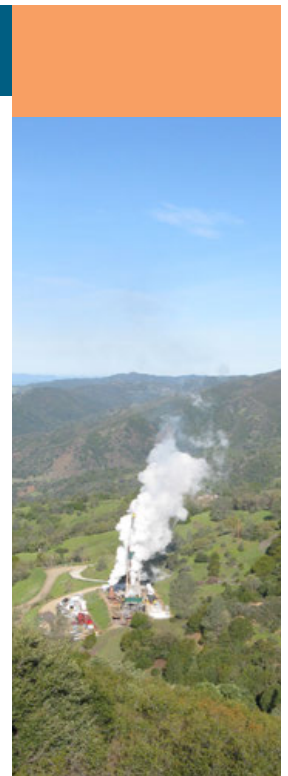
DOE's EGS Demonstration at The Geysers in California was the first in the nation to prove a commercial scale 5 MW equivalent of steam. Source: Calpine Corporation
