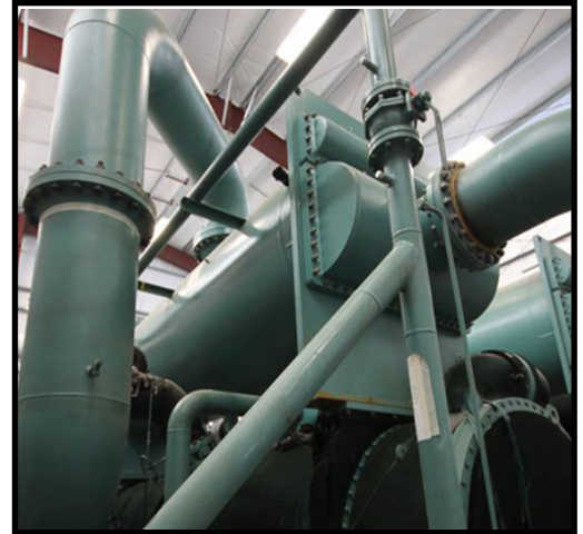
Energy Department industry partner Johnson Controls Inc. commissioned another 1.75 MW of geothermal energy at Oregon Institute of Technology in 2014. Source: Bill Goloski
