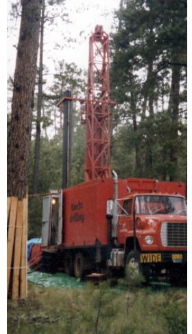
Drilling at the AltaRock EGS Newberry demonstration project in Oregon, the Energy Department's largest investment in this next generation technology. Source: GRC
