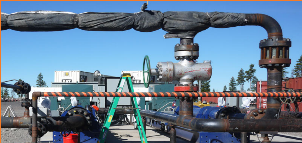
The Newberry Volcano near Bend, Oregon is one of four active EGS demonstration sites nationwide that are funded by the Geothermal Technologies Office. Source: Elisabet Metcalfe
