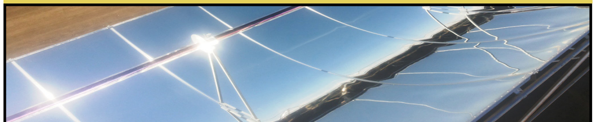
The Stillwater geothermal plant is the first hybrid solar geo facility in the nation. In 2014 Enel Green Power added 2 MW of CSP to the existing geothermal plant and solar photovoltaic field, for a total installed capacity of ~60 MW. Source: Enel Green Power North America
