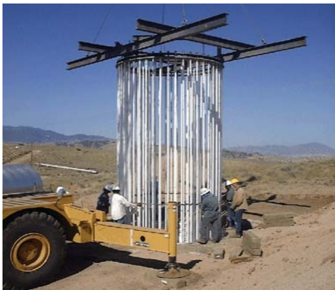
FIGURE 3.3-2 Installation of Turbine Pier Foundation (Source: Photo courtesy of RES Americas. See http://www.res-americas.com for more details.)
