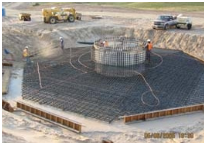
FIGURE 3.3-1 Turbine Mat Foundation under Construction (Source: Photo courtesy of RES Americas. See http://www.res-americas.com for more details.)
