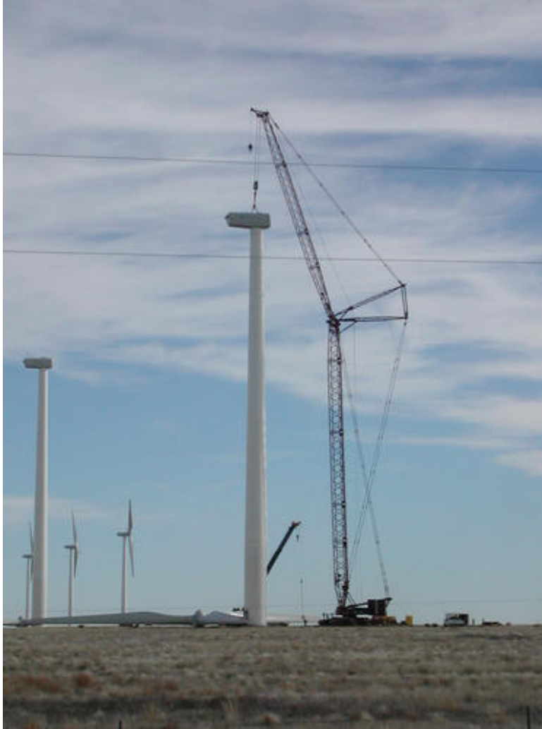
FIGURE 3.3-4 Wind Turbine Nacelle Installation at Golden Prairie Wind Farm, Lamar, Colorado (Source: NREL 2003. Photo credit: David Jager)
