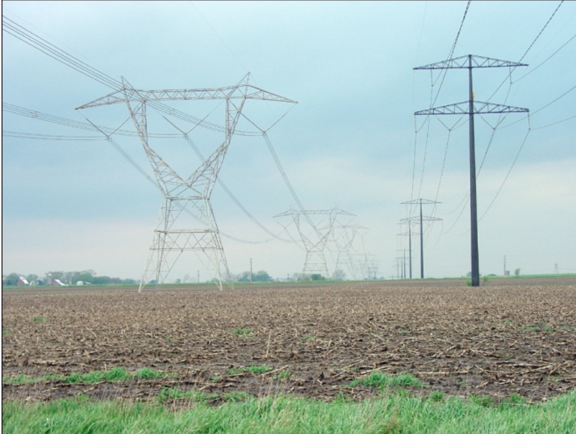
FIGURE 5.7-3 Transmission Structures: Lattice (left) and Monopole (right)
