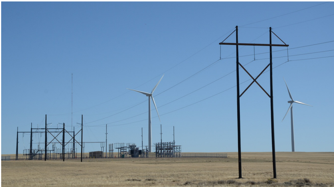
FIGURE 5.7-4 H-Frame Transmission Structure, Substation, and Guyed Meteorological Tower at Wind Facility
