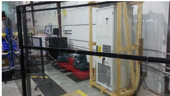
Figure 3-124: The completed dynamometer installation.
