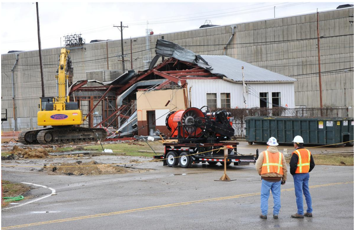
Photo 4. Demolition of the X-103 Building superstructure
