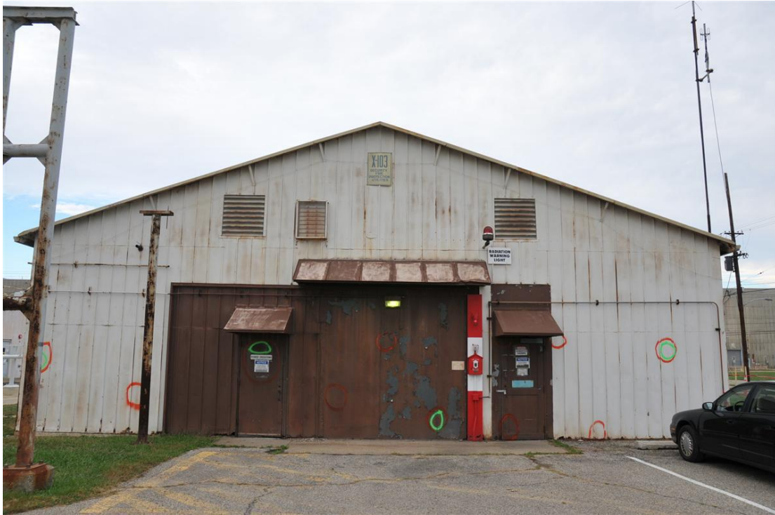
Photo 1. Front of the X-103 building facing west
