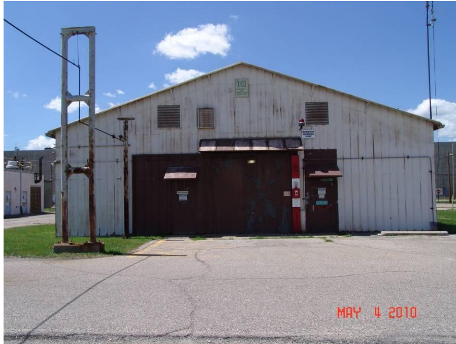
Figure 3. Photograph of front of X-103 Building facing west.
