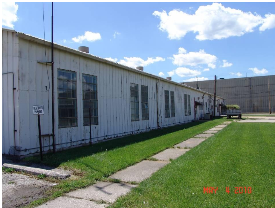
Figure 4. Photograph of north side of X-103 Building facing west.
