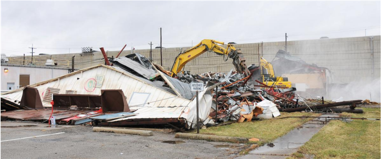
Photo 5. X-103 Building superstructure nearly demolished
