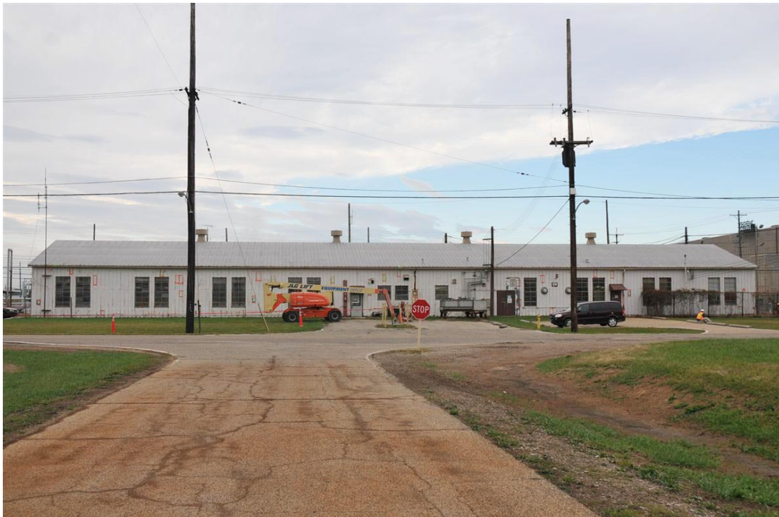
Photo 2. North side of the X-103 Building
