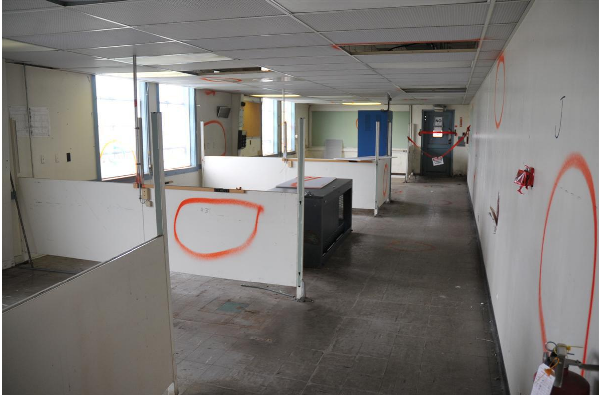
Photo 3. Interior of the X-103 Building
