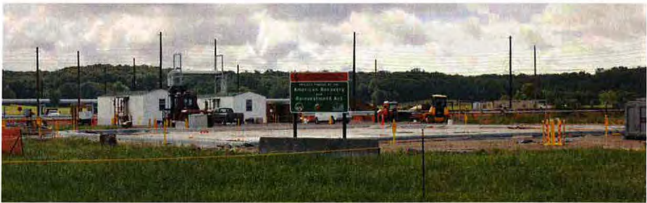
Figure 10. Photograph of the X-760 Building: northwest corner – after above-grade structure demolition
