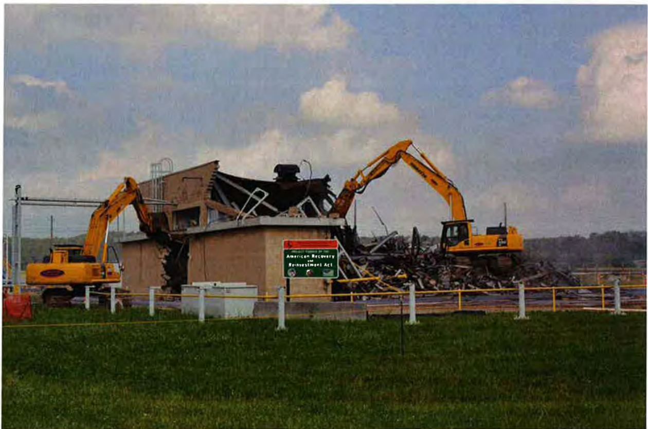
Figure 8. Photograph of the X-760 Building: northwest corner – during above-grade structure demolition
