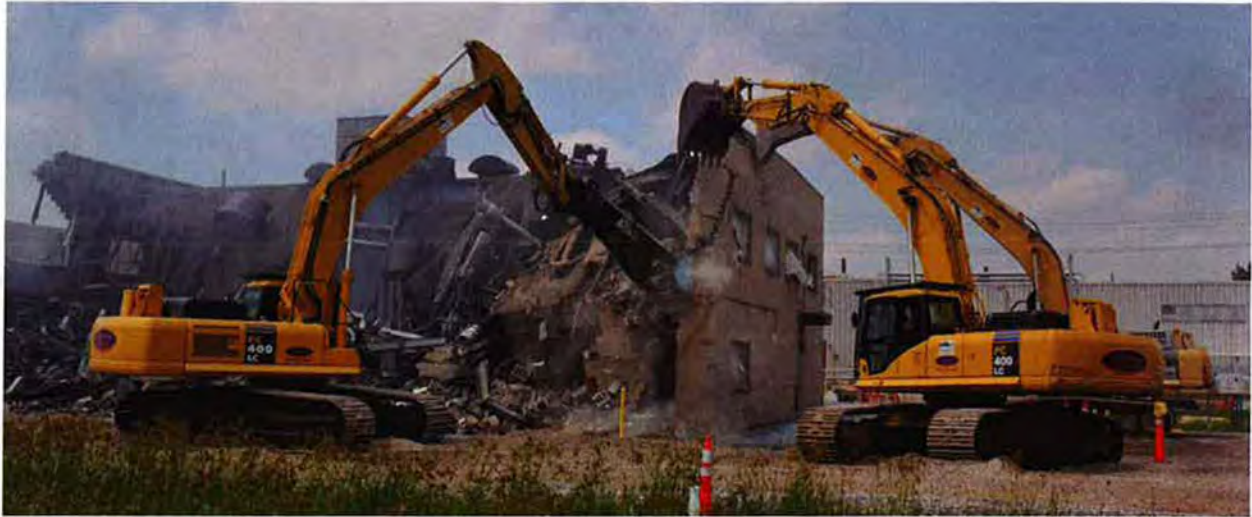
Figure 7. Photograph of the X-760 Building: south side – during above-grade structure demolition
