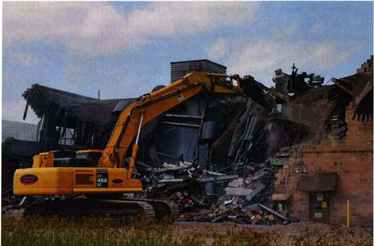
Figure 6. Photograph of the X-760 Building: south side – during above-grade structure demolition
