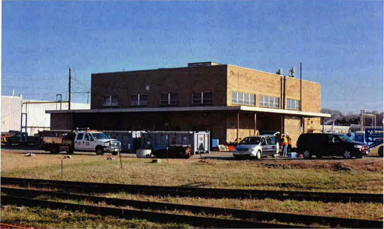
Figure 3. Photograph of the X-760 Building: southwest corner – before demolition
