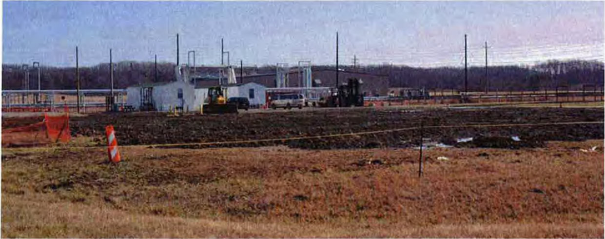
Figure 13. Photograph of the X-760 Building removal action site – during site re-contouring
