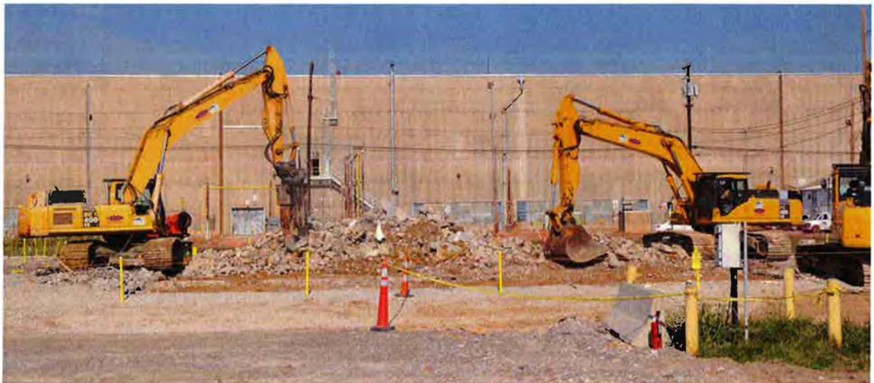
Figure 12. Photograph of the X-760 Building foundation – during concrete processing and removal
