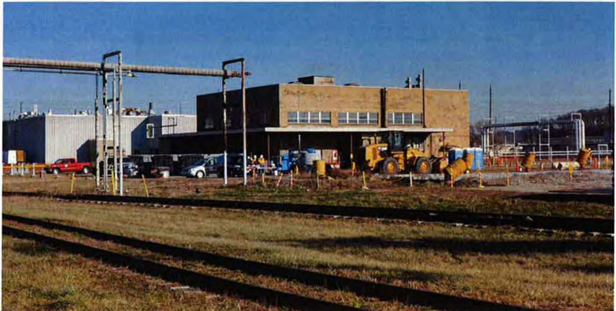
Figure 4. Photograph of the X-760 Building: south side – before demolition
