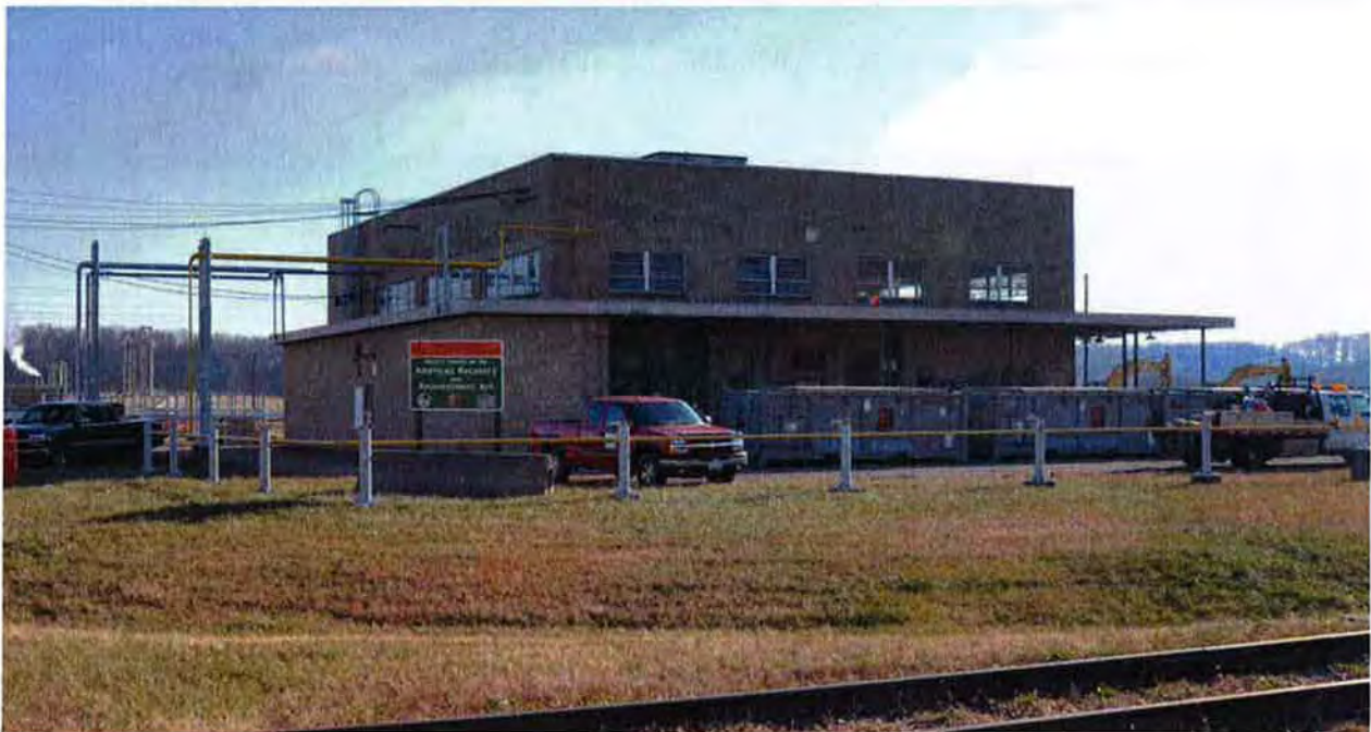
Figure 2. Photograph of the X-760 Building: west side – before demolition
