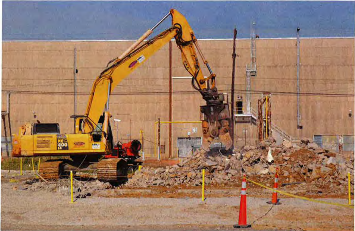
Figure 11. Photograph of the X-760 Building foundation – during concrete processing
