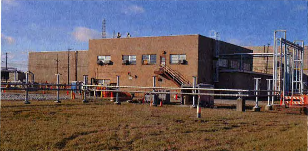
Figure 1. Photograph of the X-760 Building: east side – before demolition
