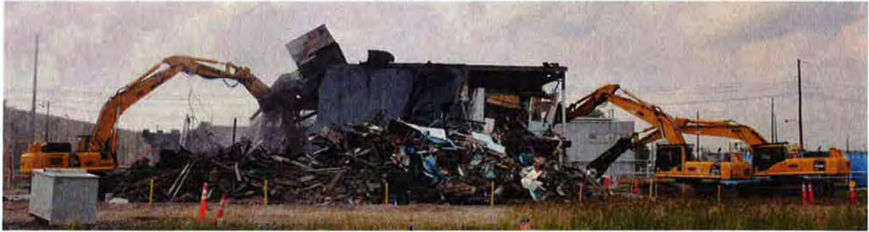
Figure 9. Photograph of the X-760 Building: south side – during above-grade structure demolition
