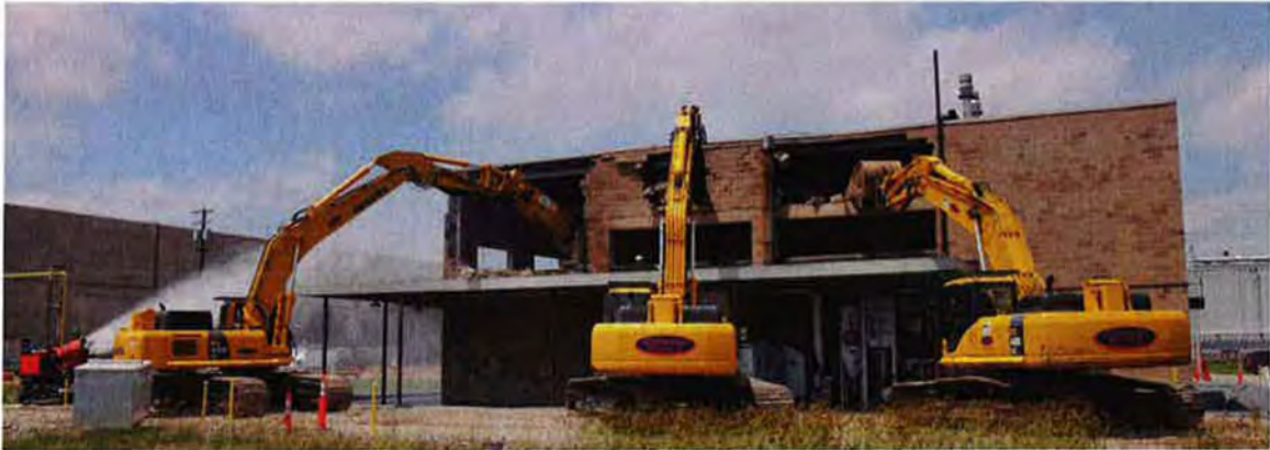
Figure 5. Photograph of the X-760 Building: south side – during above-grade structure demolition
