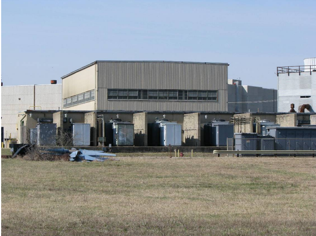
Figure A-5. Photograph of the X-633-1 Pump House – before demolition
