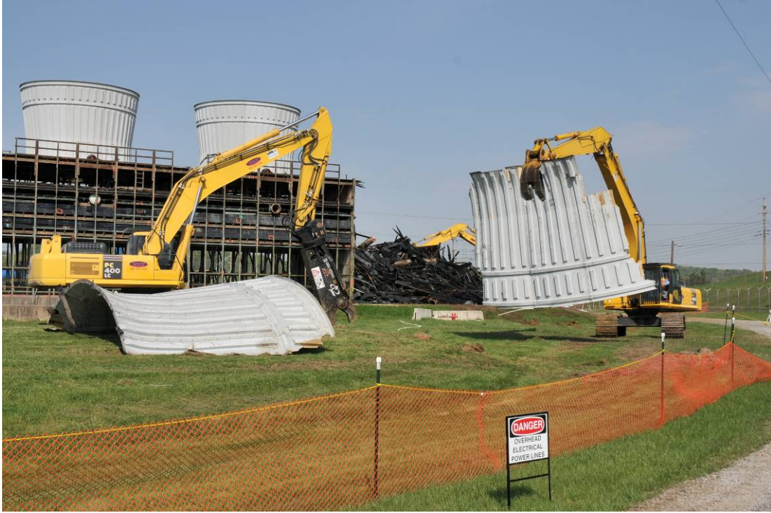
Figure A-15. Photograph of the X-633-2C Cooling Tower – during demolition
