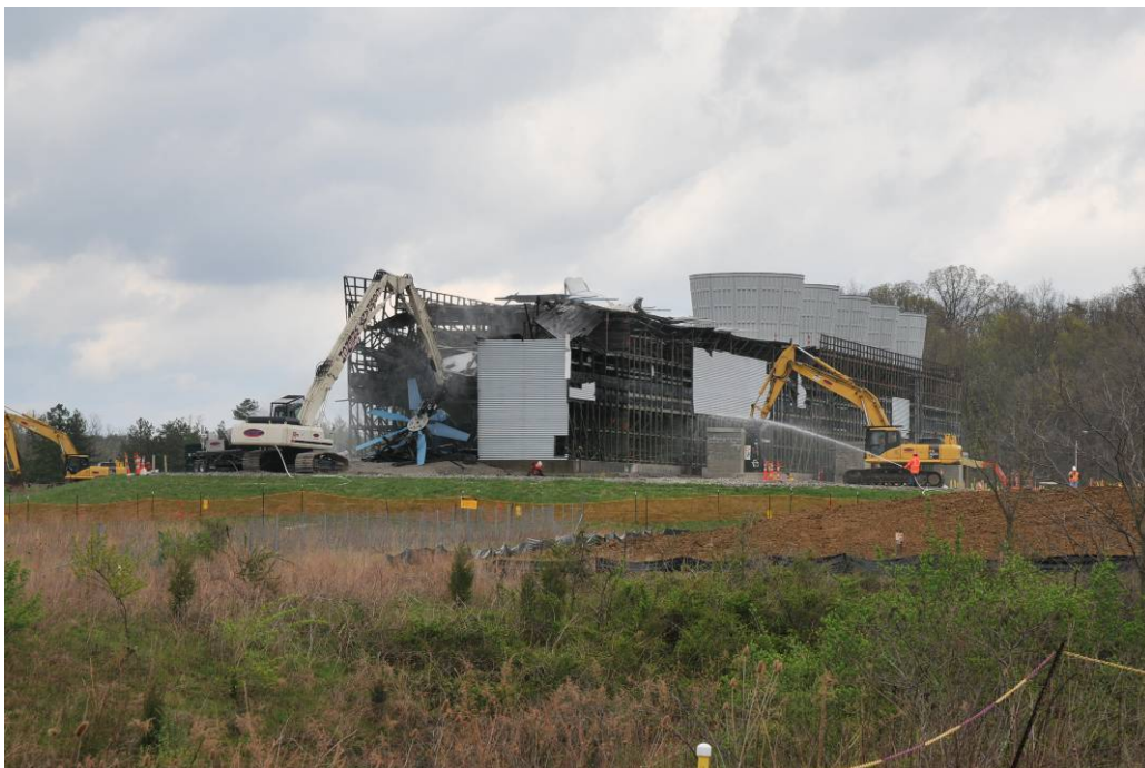
Figure A-18. Photograph of the X-633-2D Cooling Tower – during demolition
