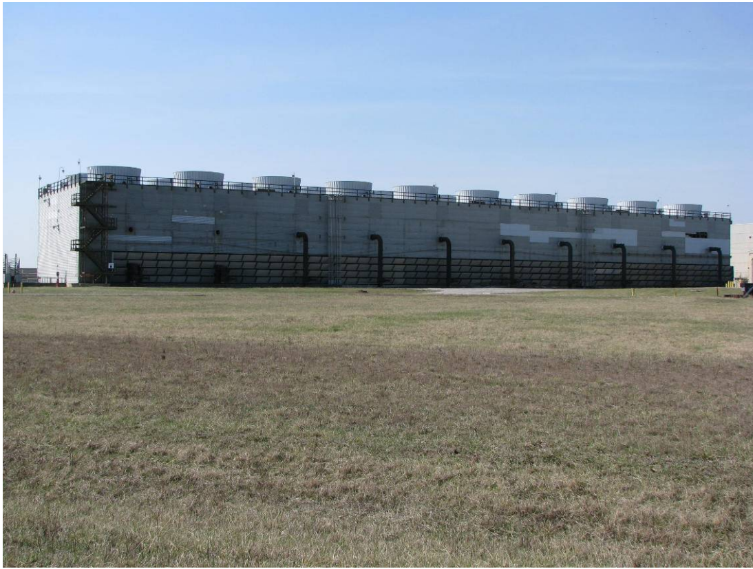
Figure A-12. Photograph of the X-633-2B Cooling Tower – before demolition
