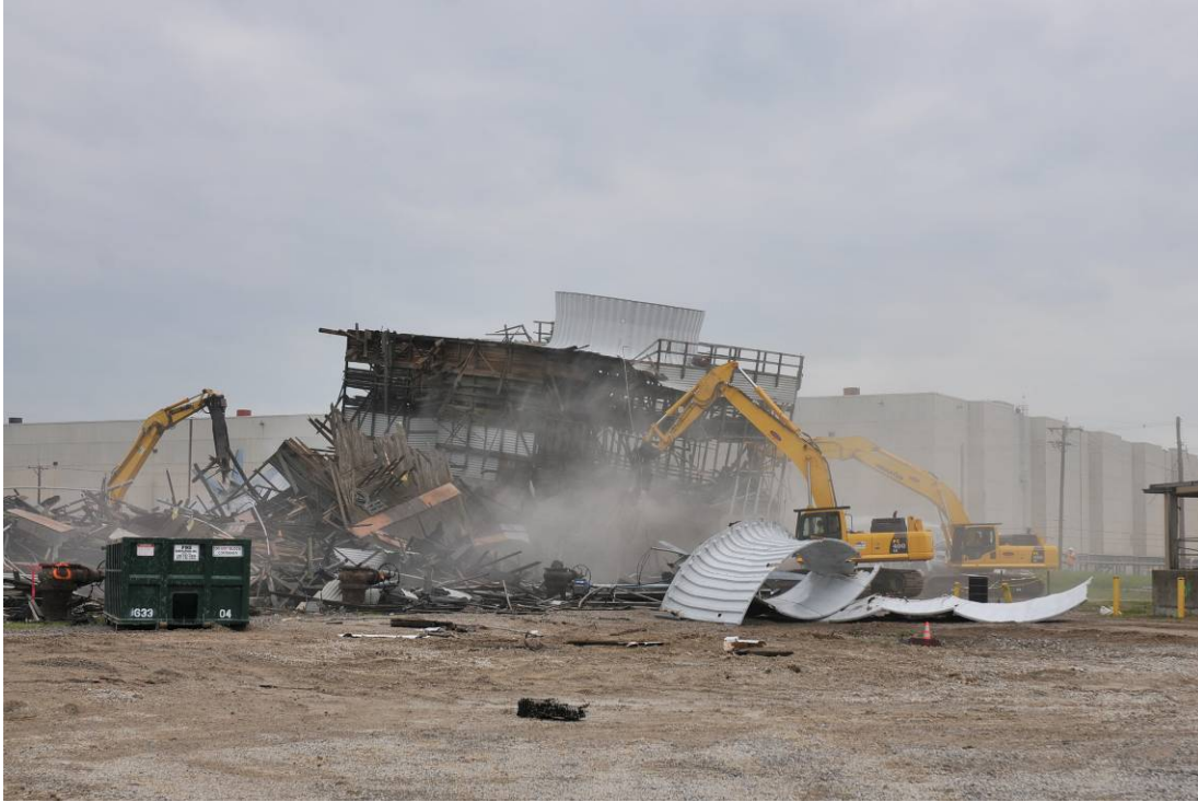
Figure A-13. Photograph of the X-633-2B Cooling Tower – during demolition
