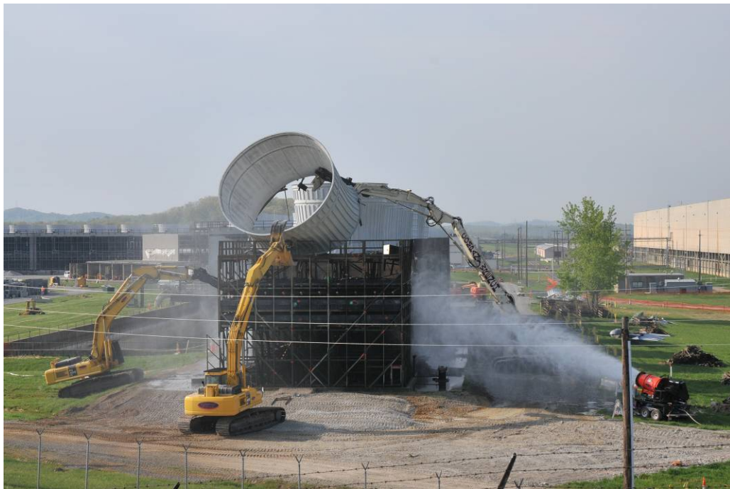
Figure A-14. Photograph of the X-633-2C Cooling Tower – during demolition
