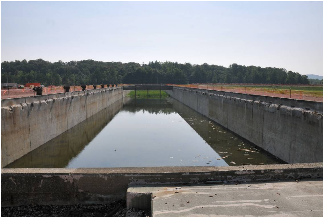
Figure A-14. Photograph of the X-633-2B Cooling Tower basin – after demolition
