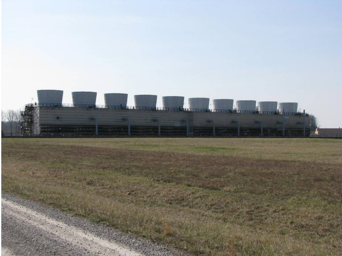
Figure A-17. Photograph of the X-633-2D Cooling Tower – before demolition
