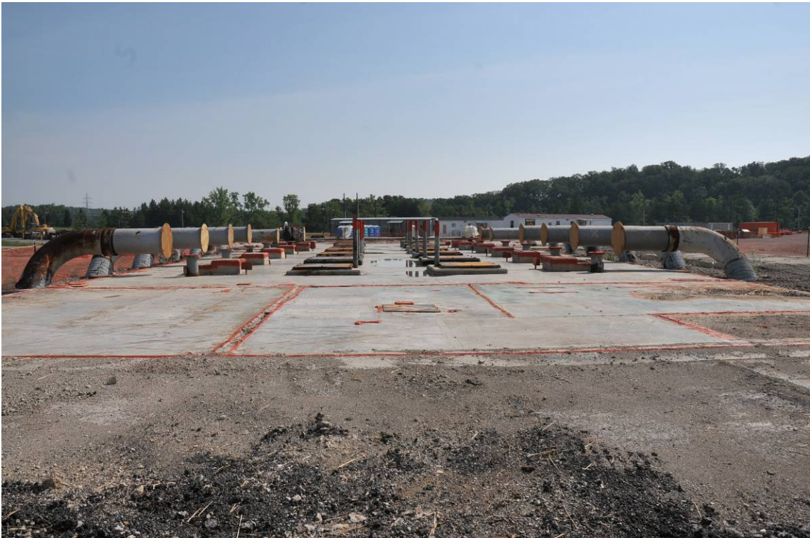
Figure A-8. Photograph of the X-633-1 Pump House – after demolition
