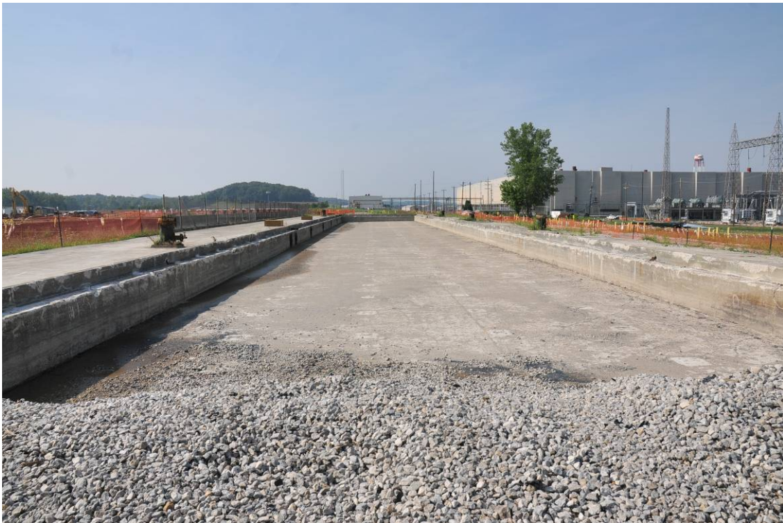
Figure A-16. Photograph of the X-633-2C Cooling Tower basin – after demolition
