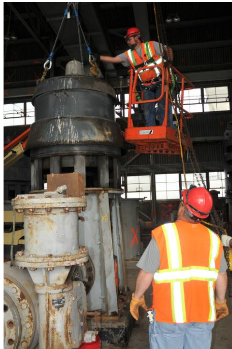
Figure A-6. Photograph of the X-633-1 Pump House – equipment removal
