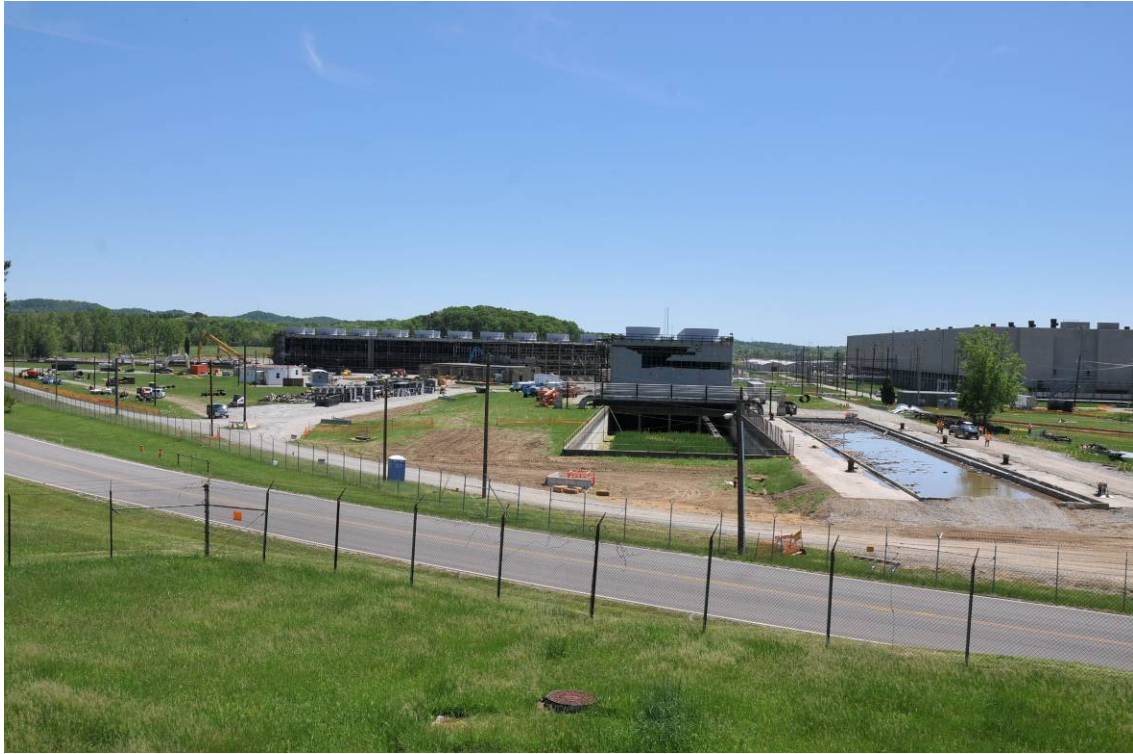
Figure A-3. Photograph of the X-633 RCW Complex – May 2010
