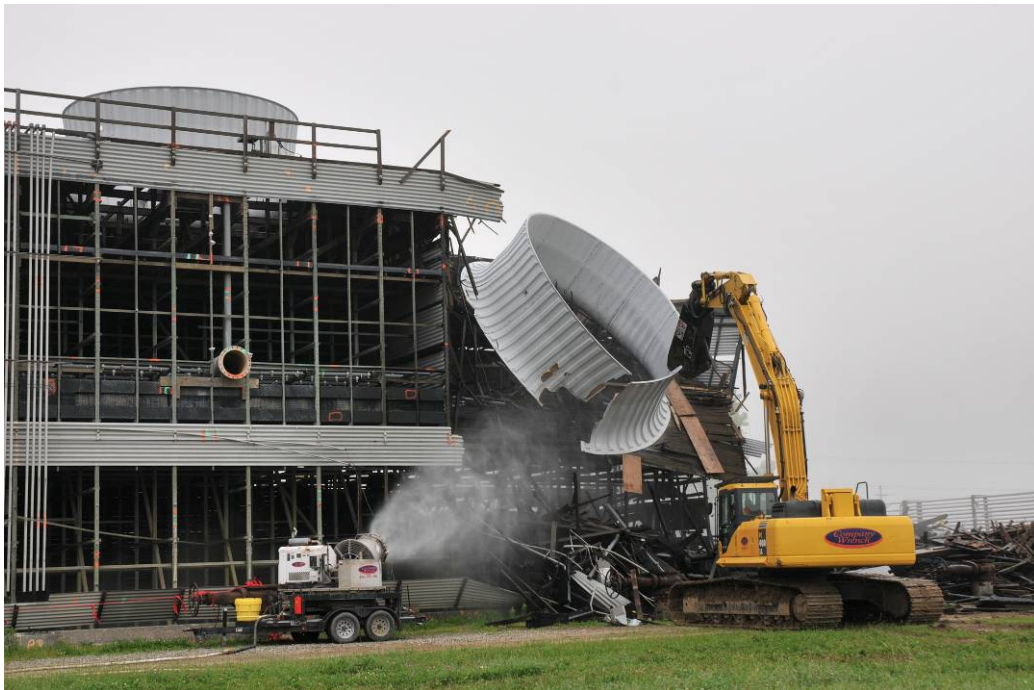
Figure A-10. Photograph of the X-633-2A Cooling Tower – during demolition
