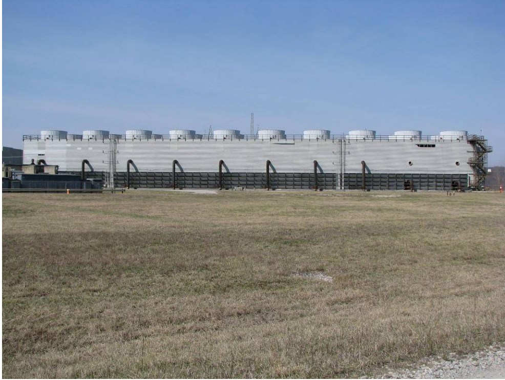
Figure A-9. Photograph of the X-633-2A Cooling Tower – before demolition
