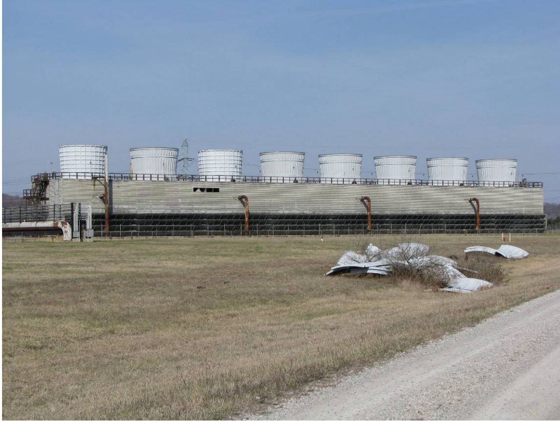
Figure A-13. Photograph of the X-633-2C Cooling Tower – before demolition
