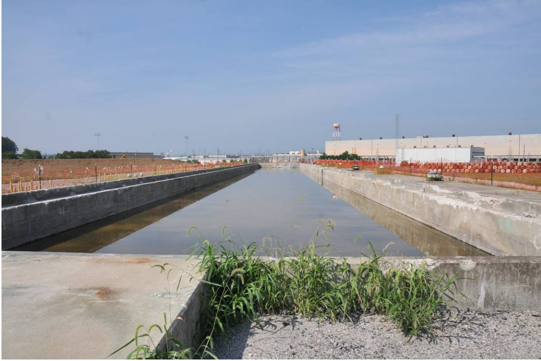
Figure A-19. Photograph of the X-633-2D Cooling Tower basin – after demolition
