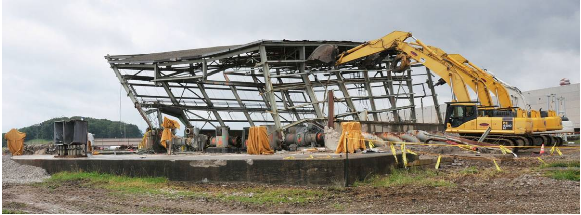
Figure A-7. Photograph of the X-633-1 Pump House – during demolition
