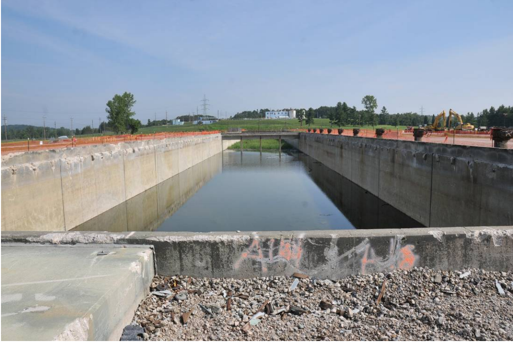
Figure A-11. Photograph of the X-633-2A Cooling Tower basin – after demolition
