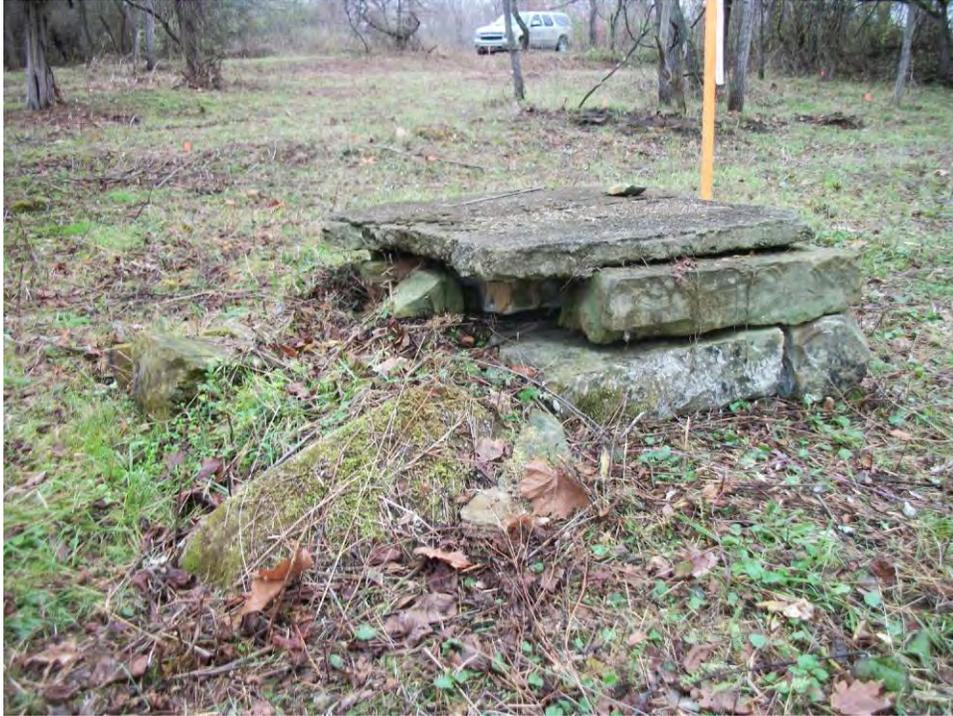
Plate 5. Raised platform foundation for stove in the house at 33PK322; facing north-northwest.
