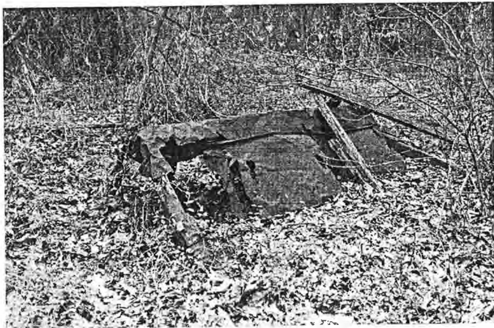
Plate 42. 33 Pk 218 (PIK-205) [Cannett Farmstead]. Woodframe and sheet metal outbuilding, facing north.
