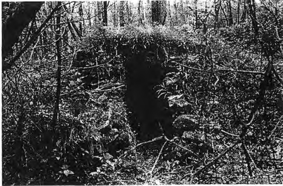
Plate 40. 33 Pk 218 (PIK-205) [Cannett farmstead]. Cement and sandstone root cellar, facing west.
