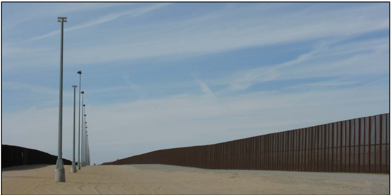
Figure 8. IGA Trial Demonstration Site - Daytime: QMH Nighthawk vs. LED Galleon-AA. The 24 ft difference in height is visible in this image. The primary fence is on the left and the secondary fence is on the right.
