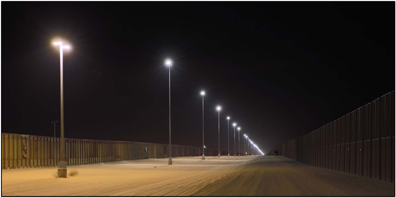
Figure 7. IGA Trial Demonstration Site - Nighttime: QMH Nighthawk vs. LED Galleon-AA. The 24 ft difference in height is visible in this image. The primary fence is on the left and the secondary fence is on the right, but is barely noticeable in this image due to the relatively low light level on the fence.
