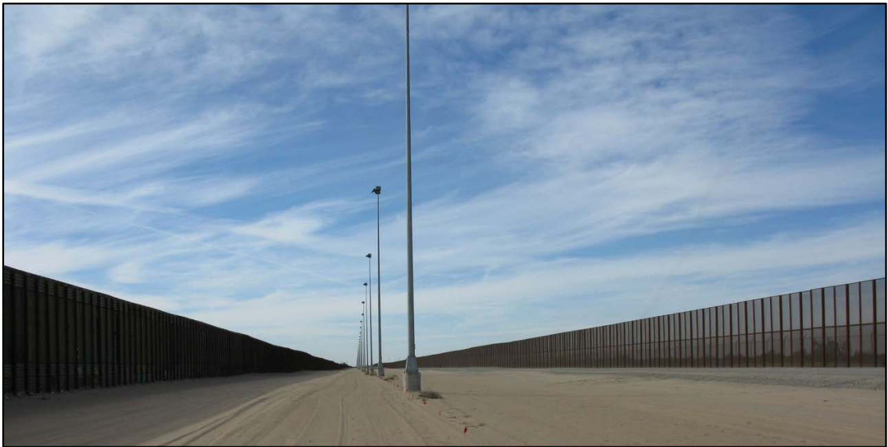
Figure 1. U.S.-Mexico Border East of San Luis POE: Area Between Primary (left) and Secondary (right) Fences. Photo taken from the east end of the 7.2 mile area, looking west. The QMH Nighthawk luminaires are mounted on the poles at a height of 64 ft.
