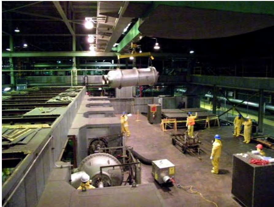
Figure 7.3. Movement of X-326 Converter
