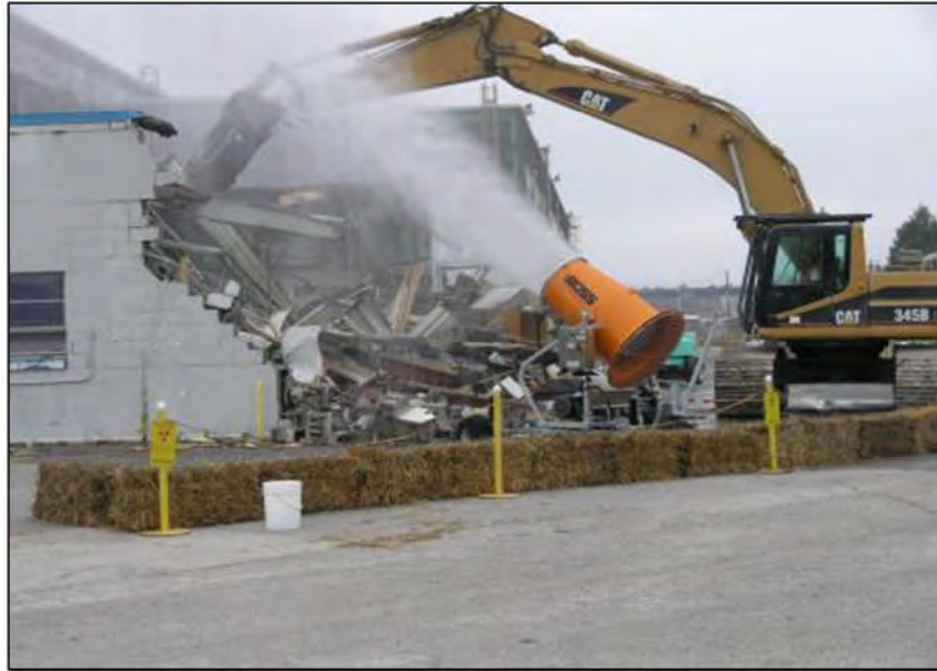
Figure 7.5. Example of Misting Technique
