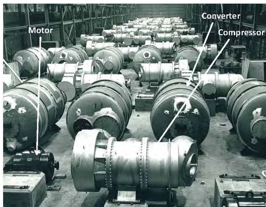
Figure A.12. Typical X-330 “00” Stage Equipment
