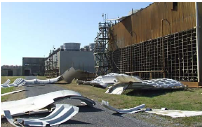
Figure 3.1. Cooling Tower Damage Sustained during 2013 Tornado
