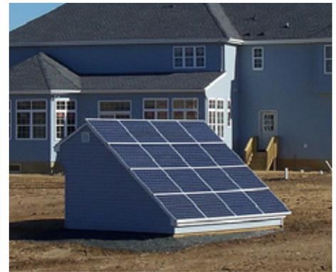
Tindall Homes installed their optional grid-tied solar photovoltaic systems on backyard garden sheds, situated for maximum solar gain. Wiring for the systems runs underground from the shed to the home's basement.
