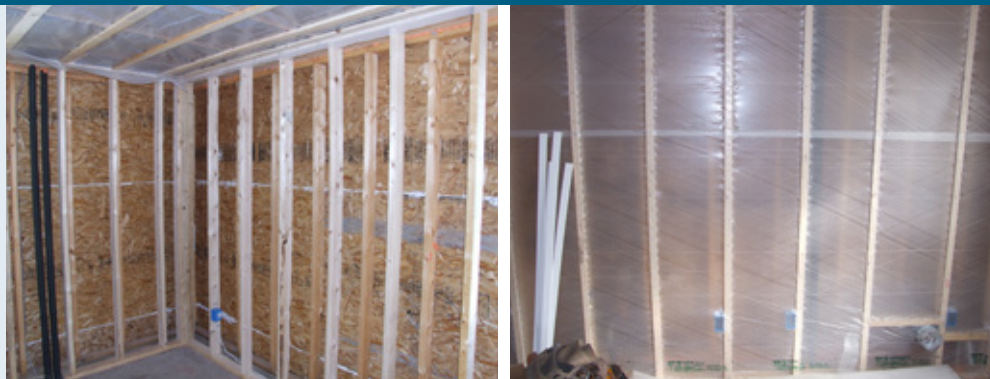
(left) The double-stud wall consists of two 2x4 16-inch on-center framed walls set 5 inches apart. (right) A vapor-permeable mesh is stapled to the inside surface of the inside wall forming a 12-inch-deep cavity to hold R-42 of dry-blown cellulose insulation.
