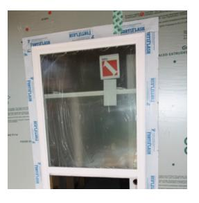
**Imagine Homes installs** double-pane, low-e, vinylframed windows. To resist water intrusion, the builder pays special attention to fully flashing windows and doors including pan flashing, and properly lapping side and top flashing. Other features that resist moisture include slab on grade foundations, fiber cement siding, and taped rigid foam exterior sheathing. Spray foam under the roof and in wall cavities helps keep hot, humid air out of the home.
