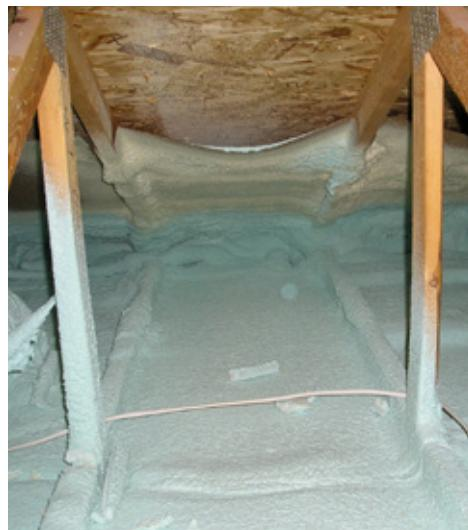
Spray foam is used to insulate and air seal the attic floor and any ducts located in the attic. The spray foam is covered with more than 12 inches of blown cellulose for the equivalent of R-49 of attic insulation.
