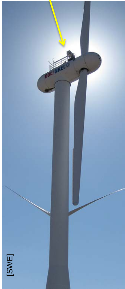
University of Stuttgart (SWE) LIDAR - CART2
