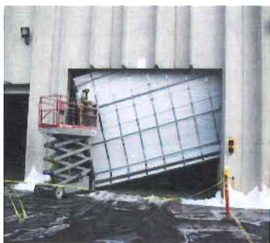
Figure 1: Example of a Roll-up Door Failure
