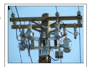
Photo of a 4kV 150 kVAR, pole-mounted, switchable capacitor bank.
