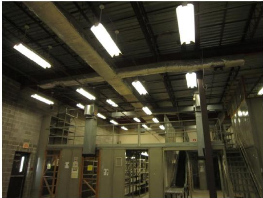
Conversion from T-12 Lamps & Mag. Ballasts to T-8 Lamps & Electronic Ballasts at Bldg. 704
