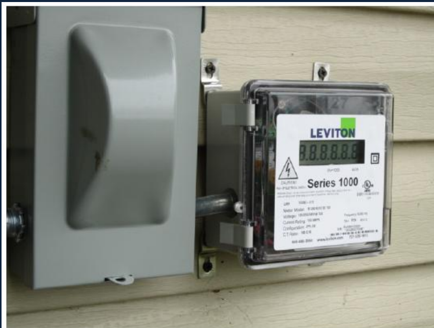
New Submeter at 127 Vinsant
