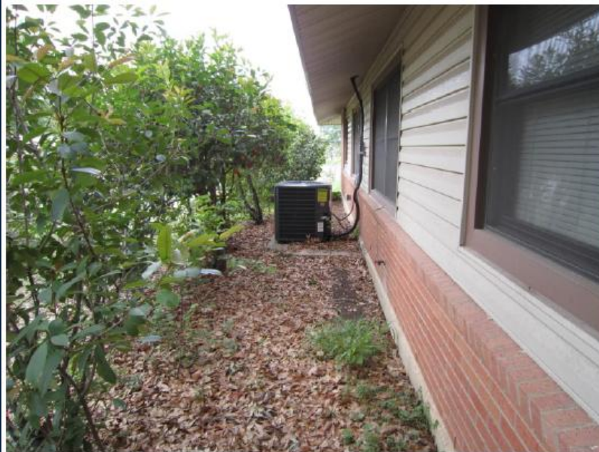
New Condenser Unit at 127 Vinsant
