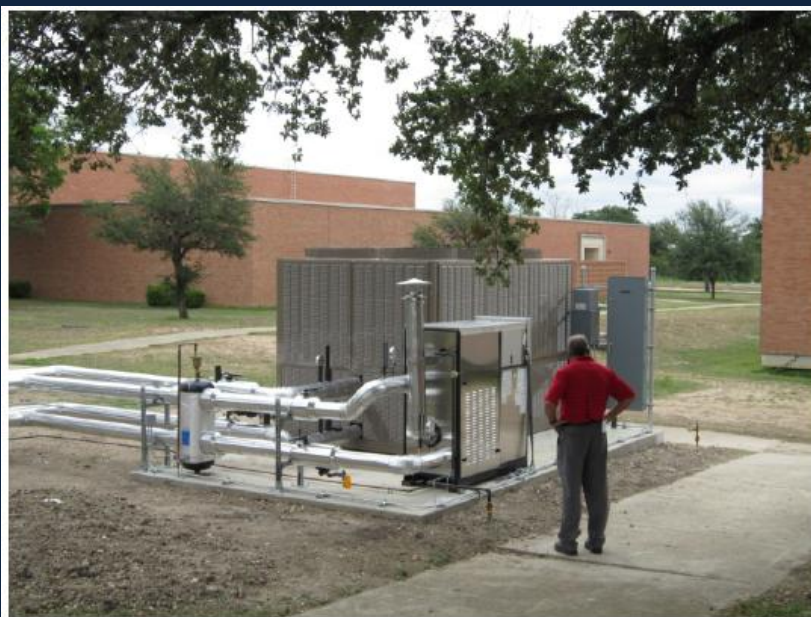
New 1,000 MBH Boiler and 100 Ton Chiller at Bldg. 155
