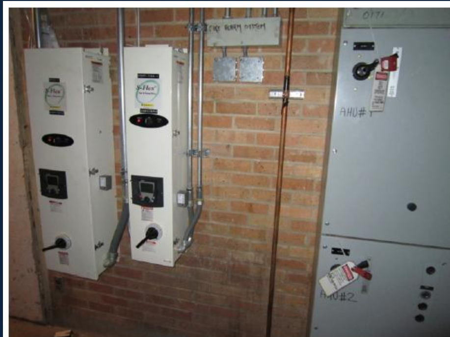
Two New AHU VFDs at Bldg. 155
