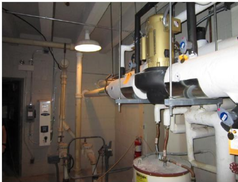
New Chilled Water Pump at Bldg. 155
