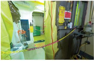
and the non-airborne contamination area. Real time air monitoring has been added in the Warm Shop and the Warm Gang Valve Corridor airlock. Lastly, a scoop/ventilation duct is used during the opening and resizing of the waste that is directed into the canyon exhaust.
